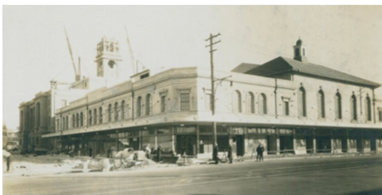
Builders put the finishing touches on Civic Theatre as work progressed on City Hall's clocktower.
