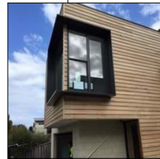
ALUMINIUM SHROUD AROUND BALCONY OPENING
