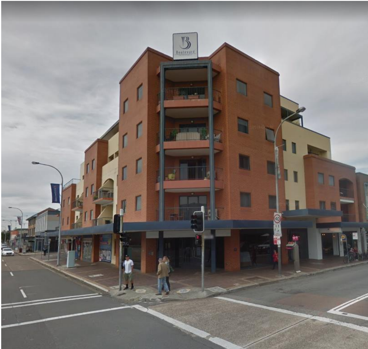
Plate 1: View of the site looking east. Source: Google Maps.
