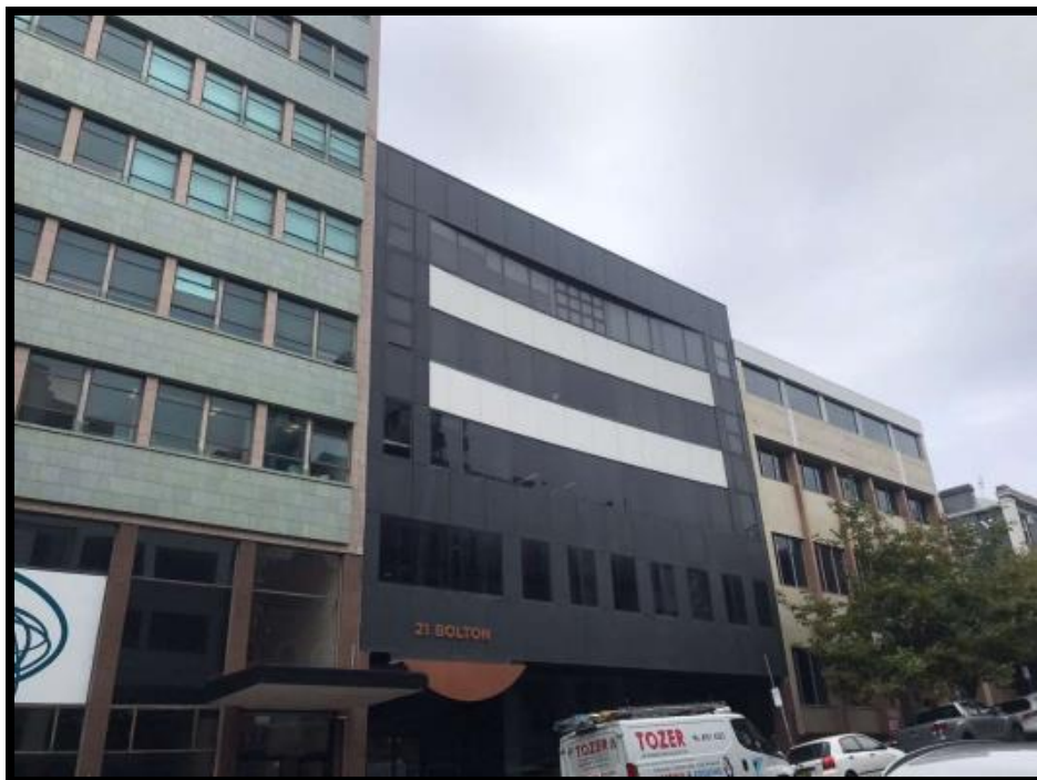
Figure 1 – View of the site from Bolton Street, facing north-east.
