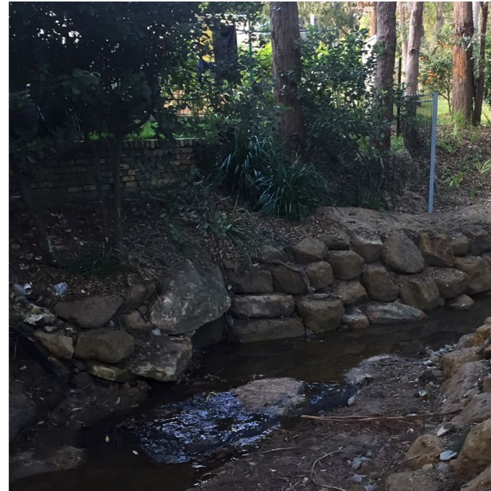
Sygna Close Rankin Park, nature-based solutions in creek rehabilitation protecting properties and promoting biodiversity
