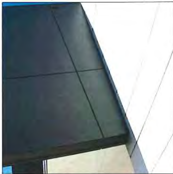
WALL CLADDING 4 - (FC) Hardies Scyon™ Matrix™ cladding
