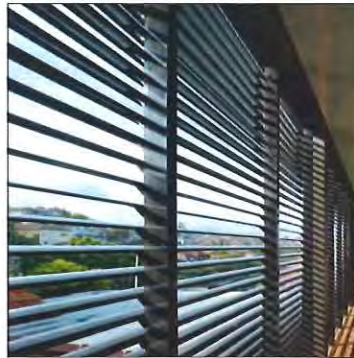
EXTERNAL LOUVRES - (TIM) Adjustable timber louvres
