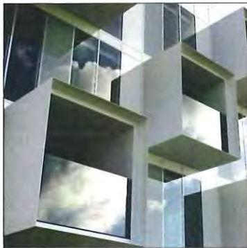
WINDOW AWNINGS Powdercoated 'white' mild steel
