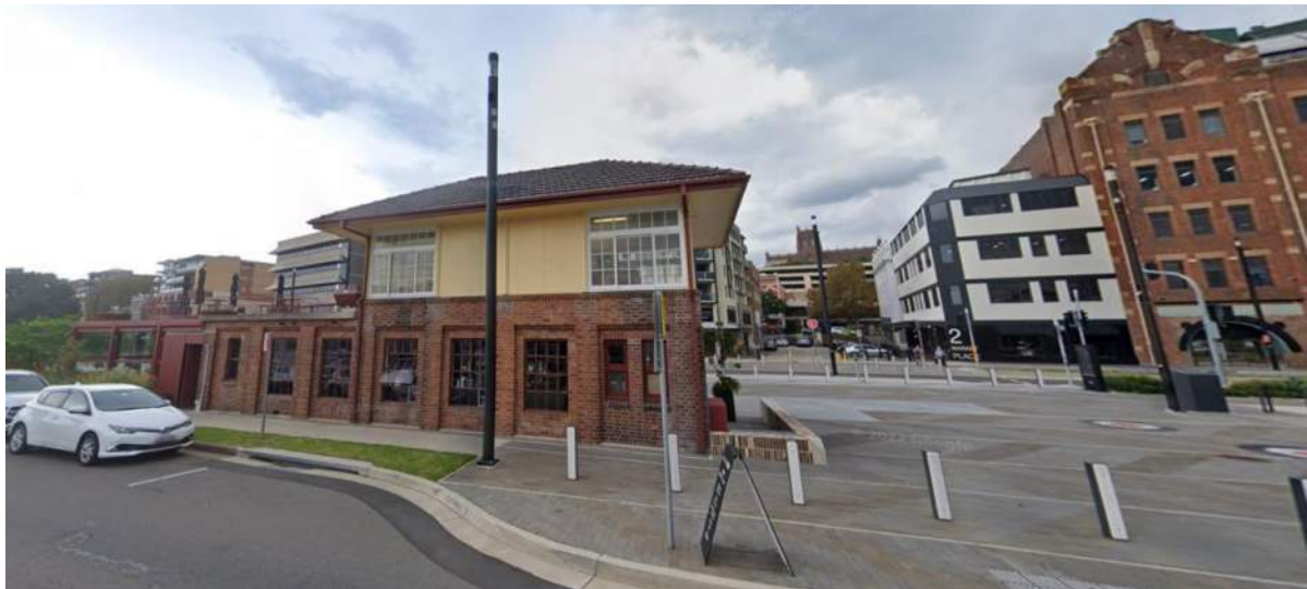
Figure 54: Newcastle Signal Box at 155 Wharf Road, Newcastle with the tower of Christ Church Cathedral in background (Source: Google Streetview)
