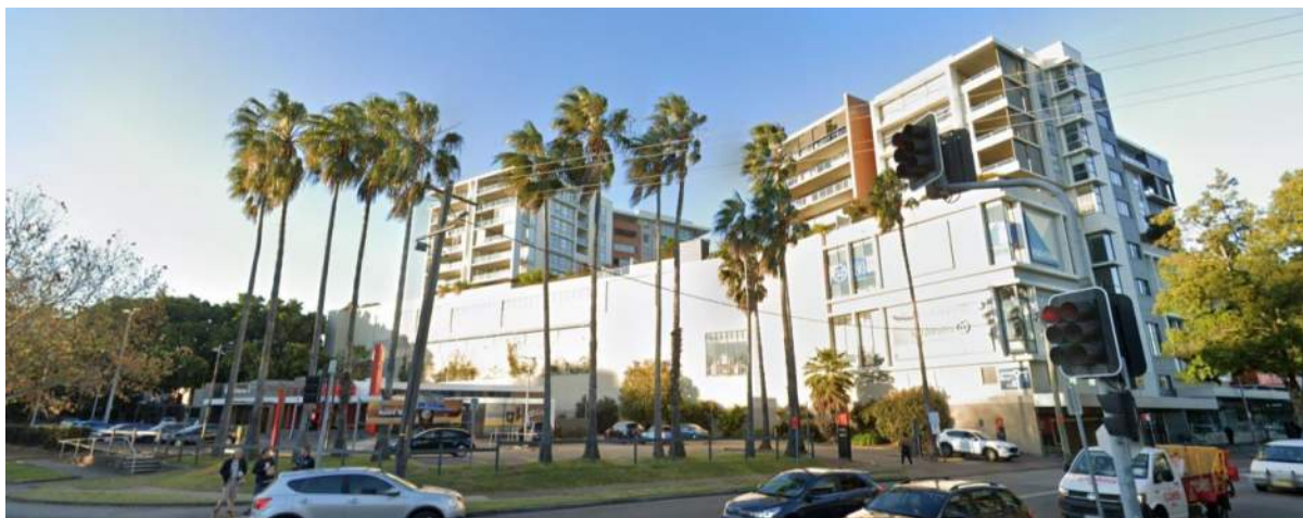
Figure 108: 19 and 21 Steel Street, Newcastle West (Source: Google Streetview)
