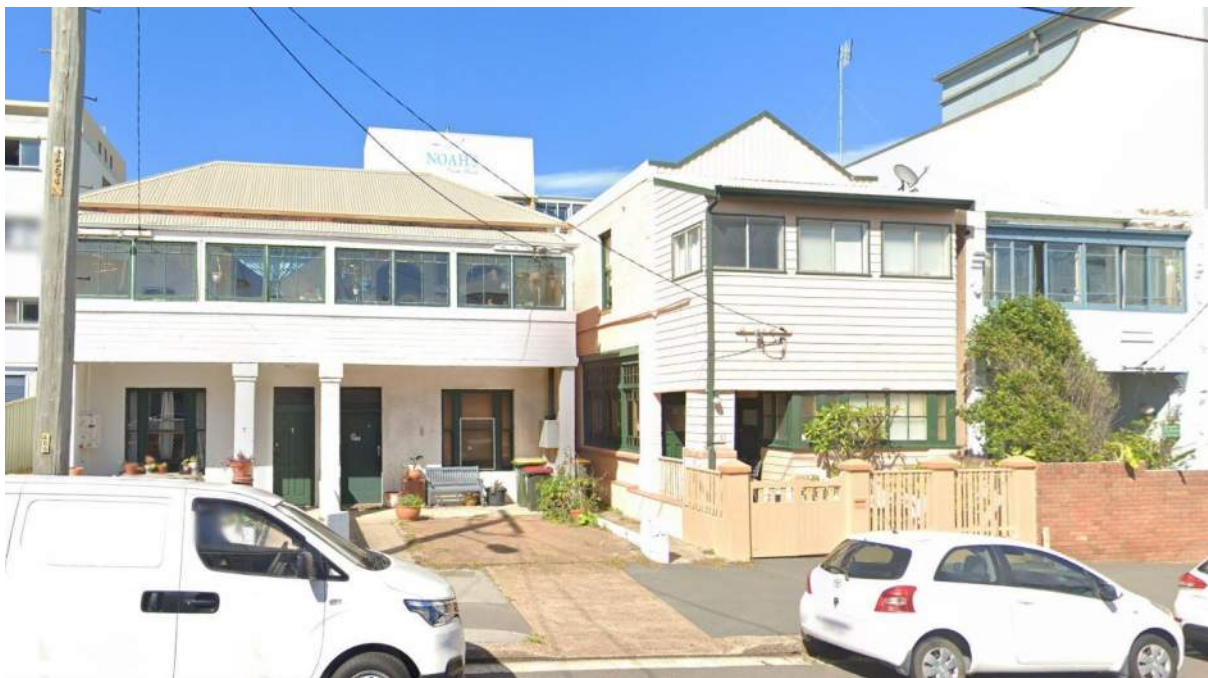
Figure 41: 7 to 15 (odd numbers) Scott Street facing south (Source: Google Streetview)
