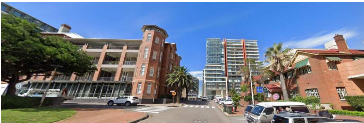
Figure 56: Newcastle Hospital North Wing at 2 Ocean Street and Former Nurses' Home (Royal Newcastle Hospital - The Club Building) at 30 Pacific Street, Newcastle (Source: Google Streetview)
