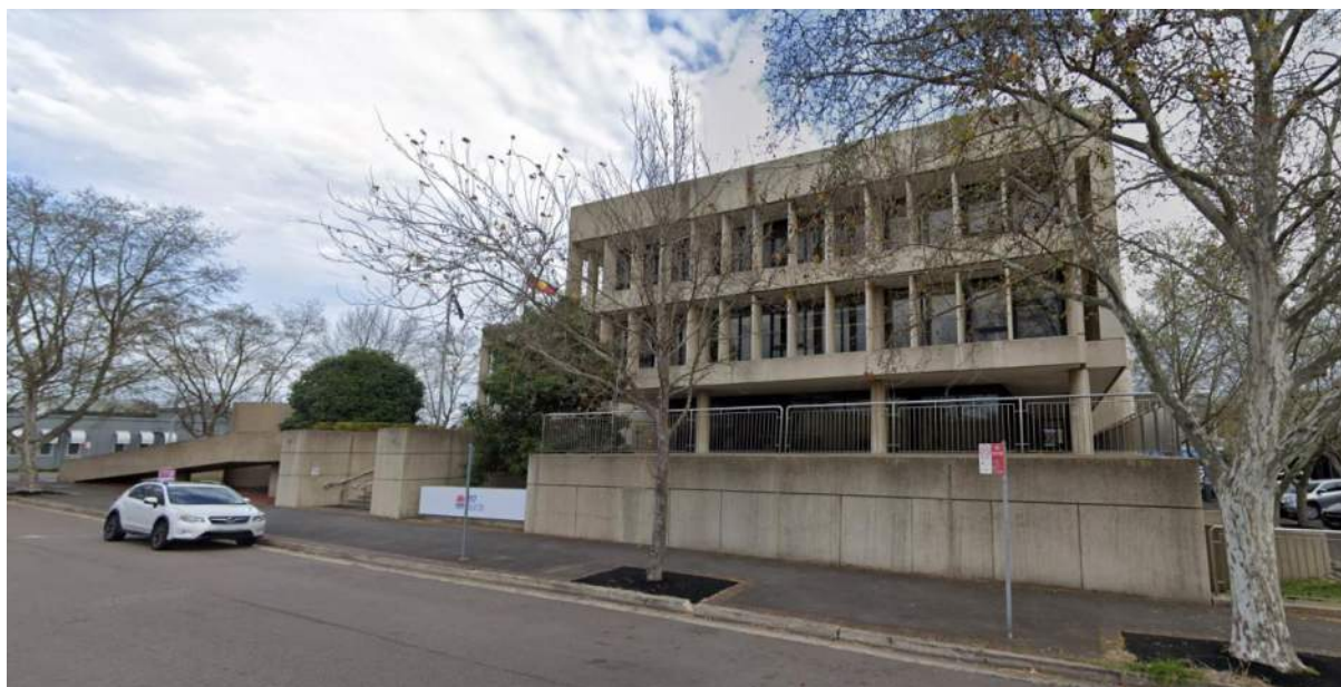
Figure 115: 117 Bull Street, Newcastle West (Source: Google Streetview)
