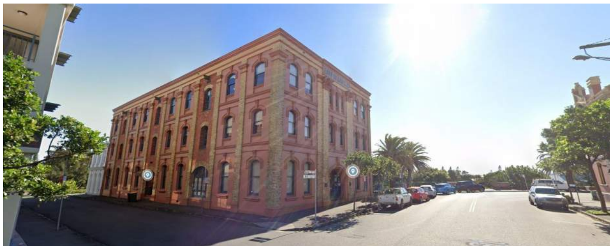
Figure 30: Earp Gillam Bond Store at 16 Telford Street, Newcastle East (Source: Google Streetview)
