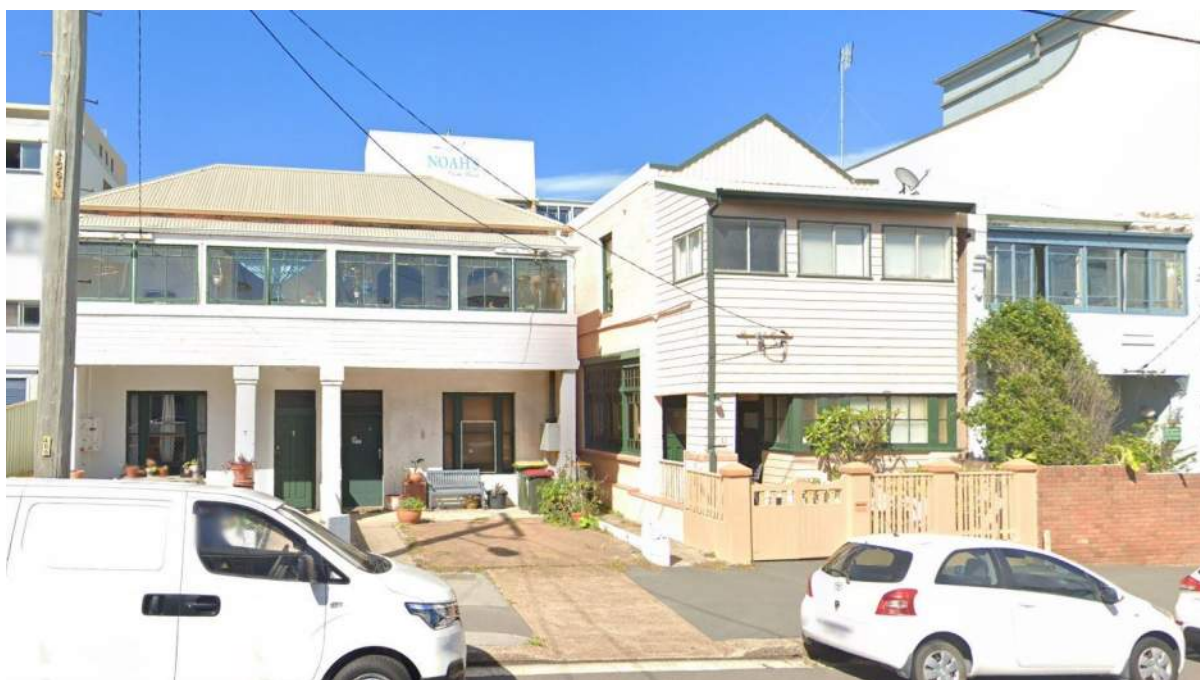
Figure 41: 7 to 15 (odd numbers) Scott Street facing south (Source: Google Streetview)
