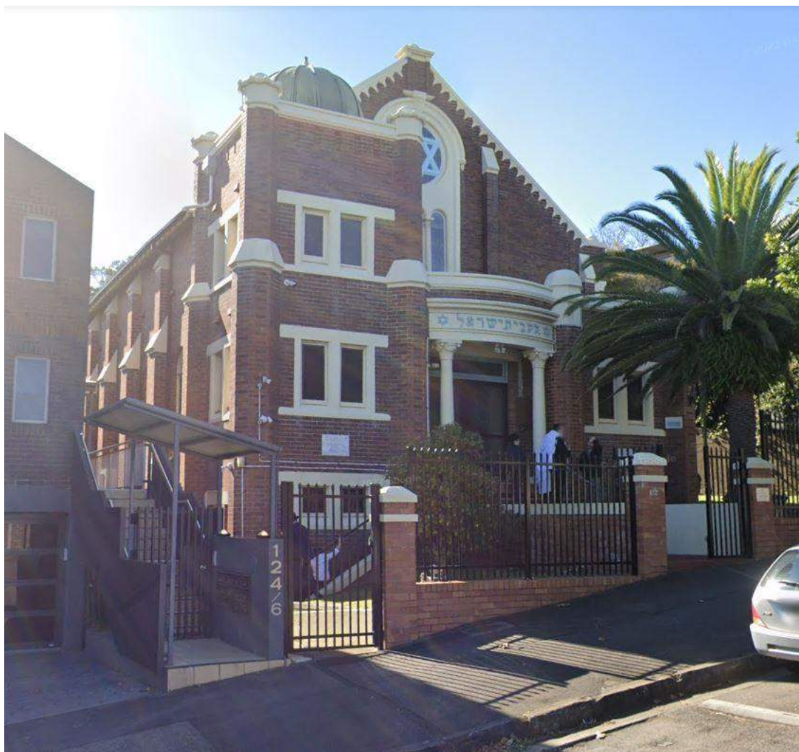
Figure 89: the Newcastle Synagogue at 122 Tyrell Street, The Hill (Source: Google Streetview)
