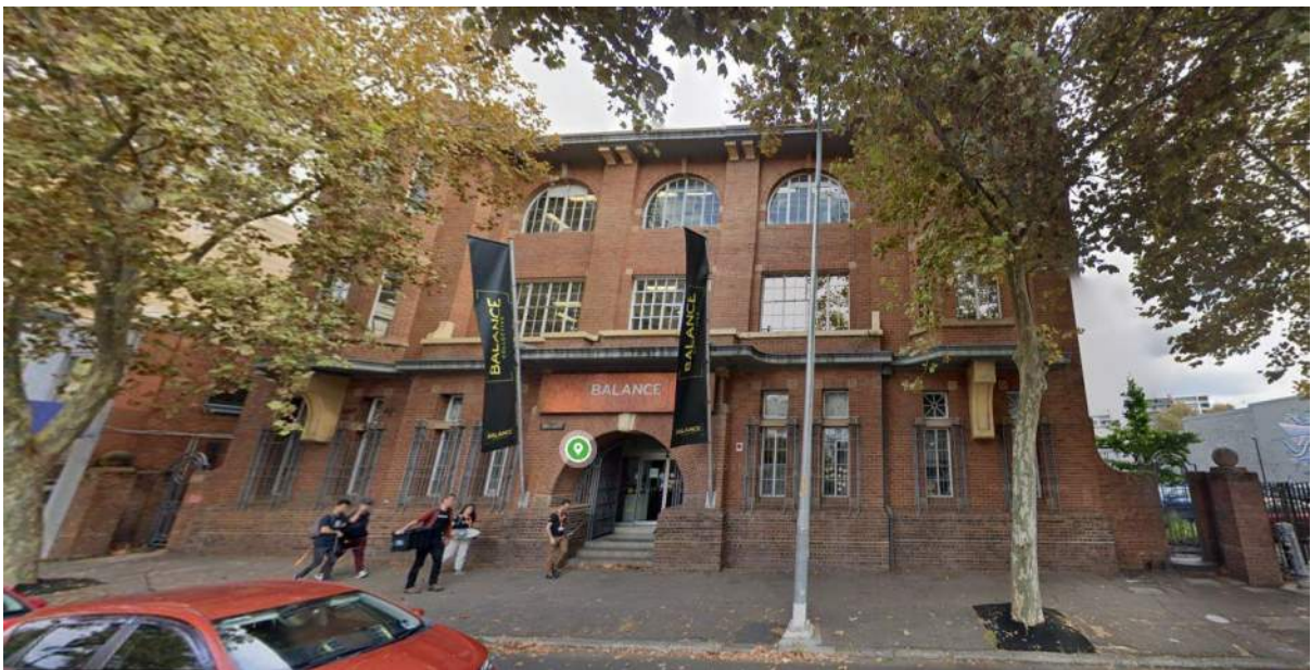
Figure 102: the Hunter Water Board Building at 591-595 Hunter Street, Newcastle West (Source: Google Streetview)
