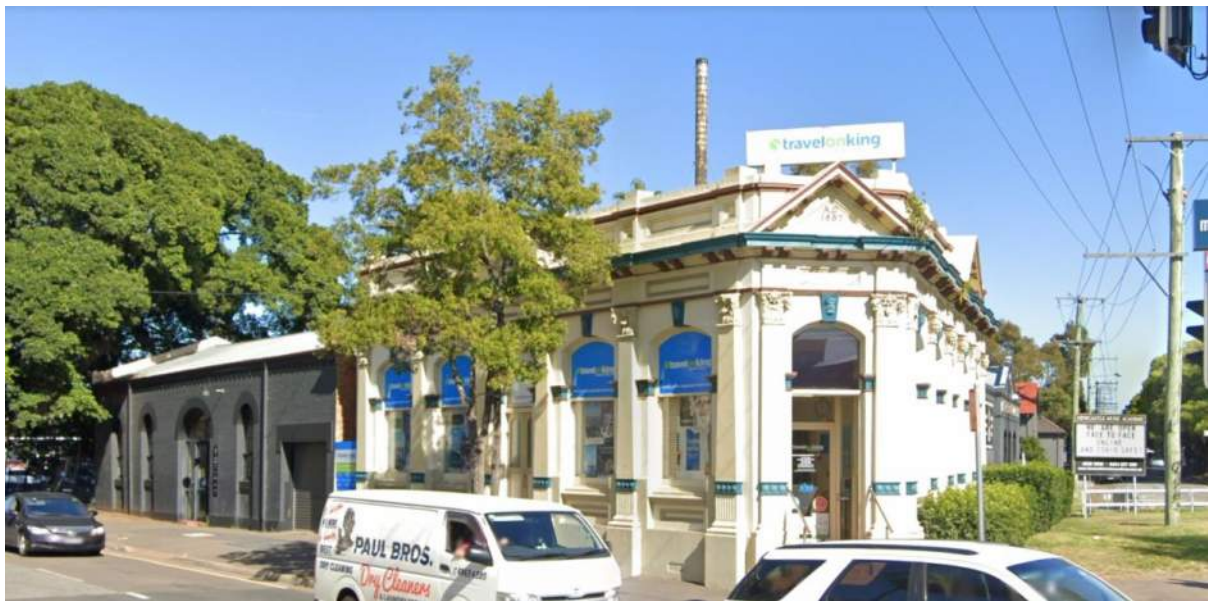
Figure 114: Former Gasworks Office at 461 King Street, Newcastle West (Source: Google Streetview)
