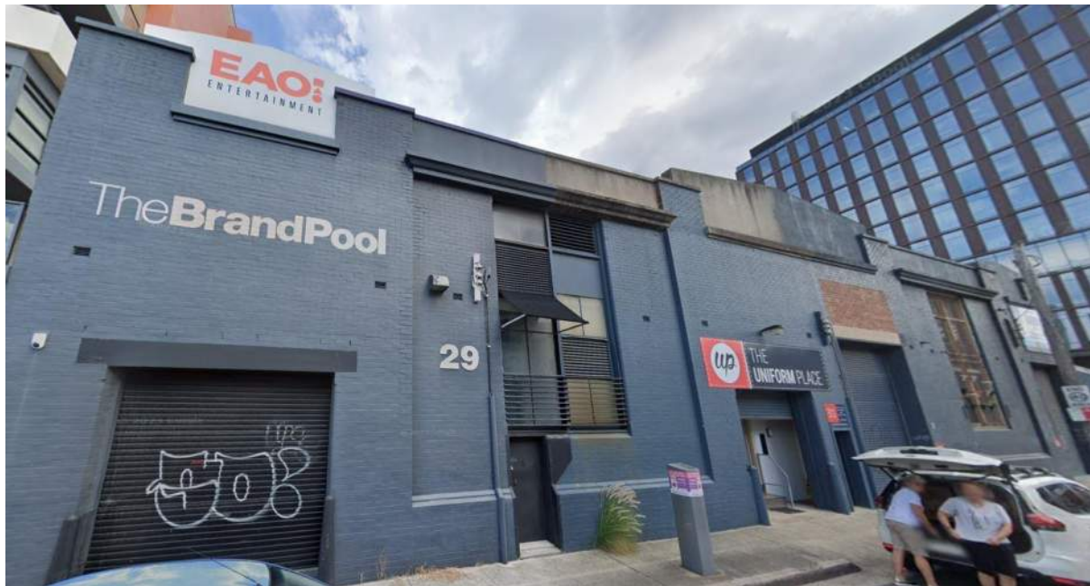
Figure 139: 29 and 31 Beresford Street, Newcastle West (Source: Google Streetview)
