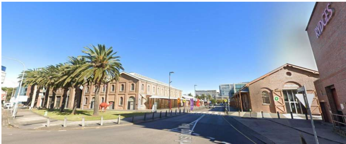
Figure 76: Civic Railway Workshops (Source: Google Streetview)
