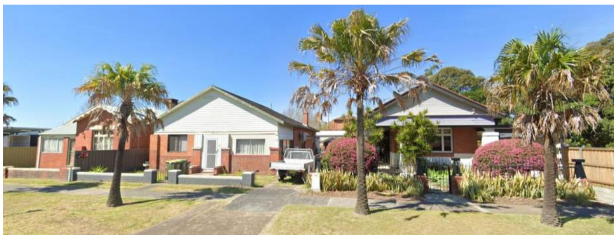
Figure 128: 1, 3 and 5 Selma Street, Newcastle West (Source: Google Streetview)
