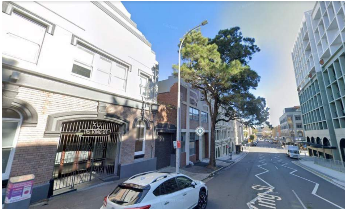
Figure 63: 115 King Street, Newcastle facing west (Source: Google Streetview)
