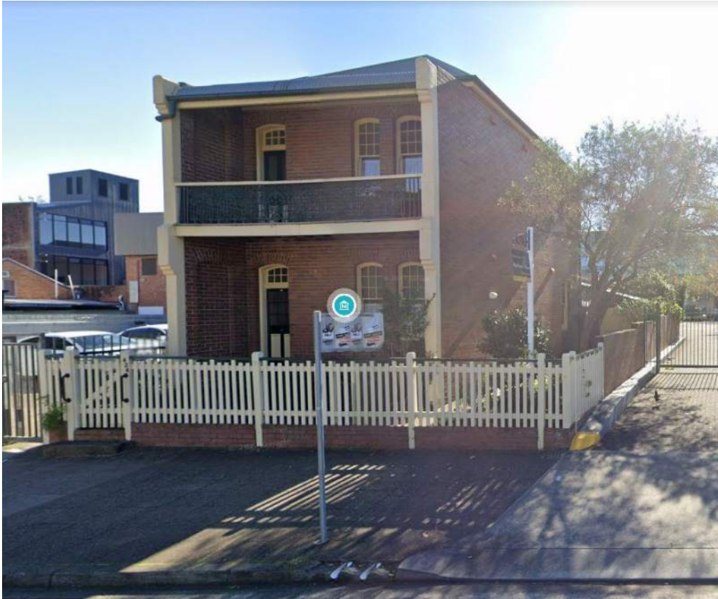
Figure 103: Miss Porter's House at 434 King Street, Newcastle West (Source: Google Streetview)
