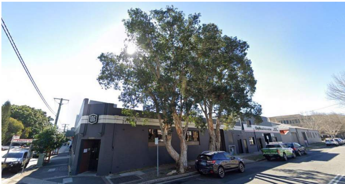
Figure 112: 106 Parry Street, Newcastle West facing north (Source: Google Streetview)
