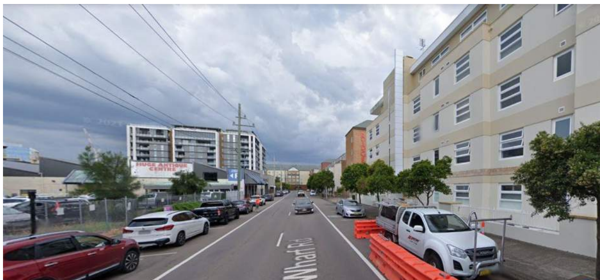
Figure 81: 317 and 304 Wharf Road, Newcastle facing west (Source: Google Streetview)
