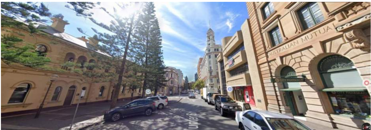
Figure 51: 90 and 55 Hunter Street, Newcastle - view east towards T&G Mutual Life Assurance Building at 45 Hunter Street, Newcastle (Source: Google Streetview)
