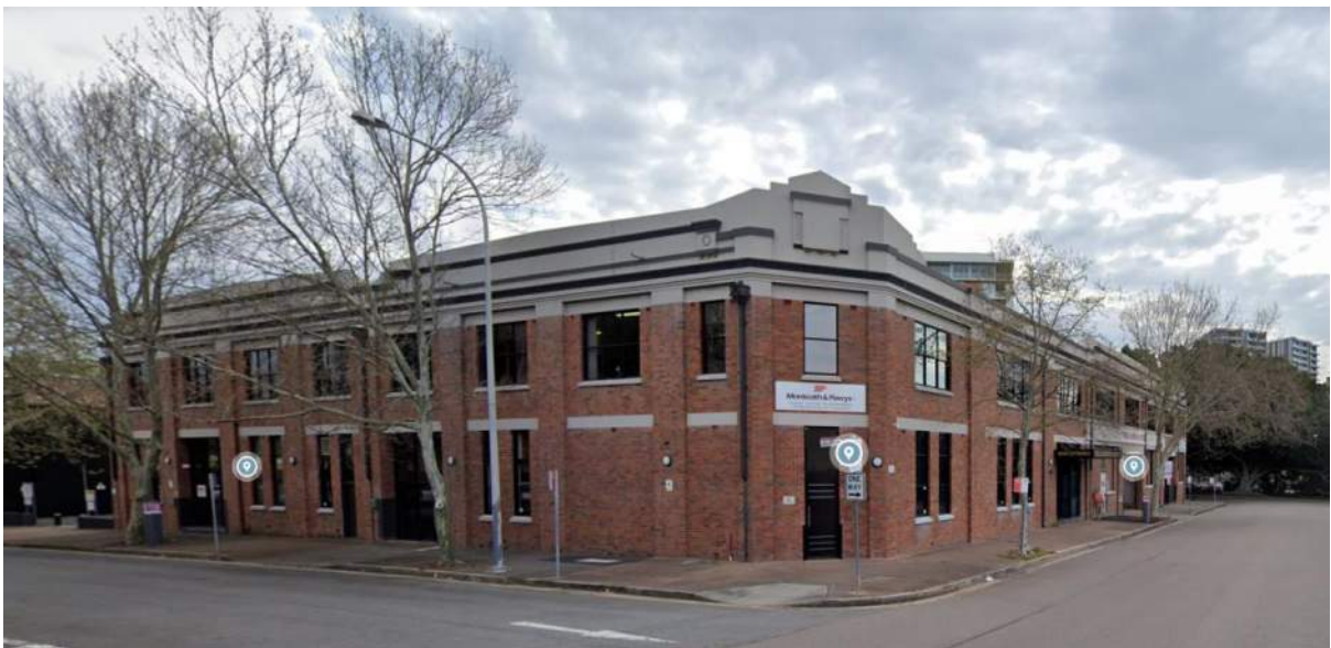
Figure 116: 125 Bull Street, Newcastle West (Source: Google Streetview)
