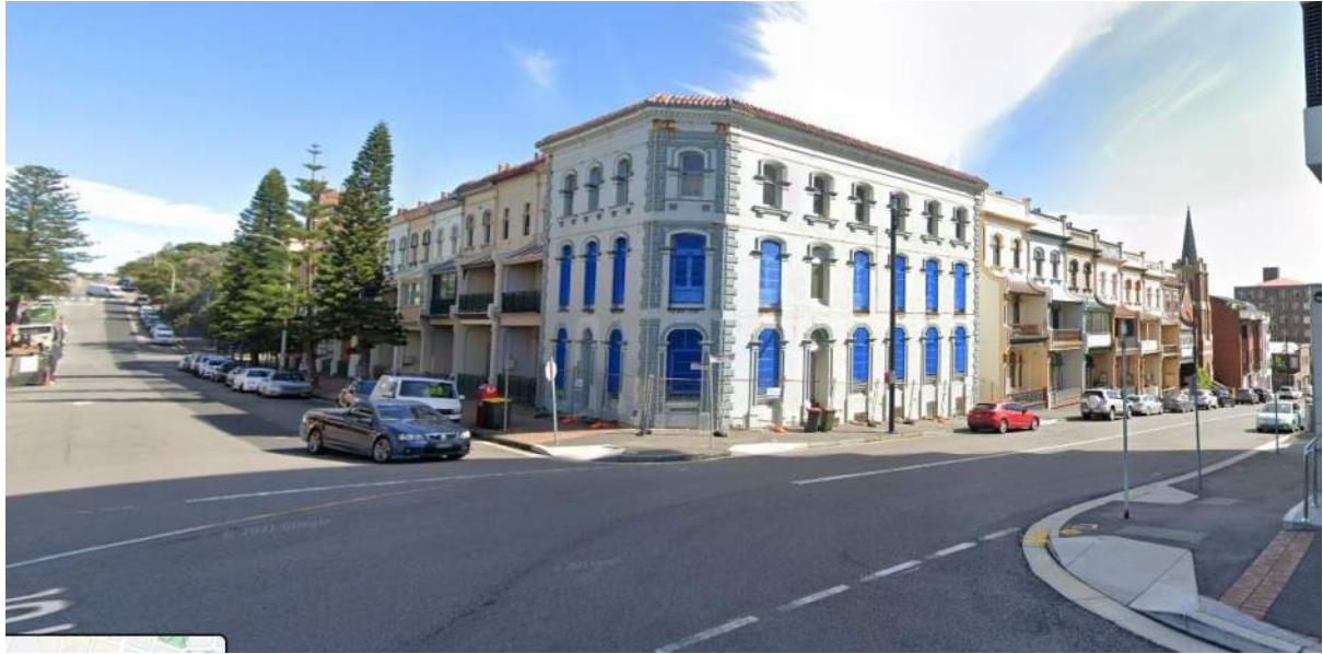
Figure 53: Church and Watt Street Terraces Group, Newcastle (Source: Google Streetview)
