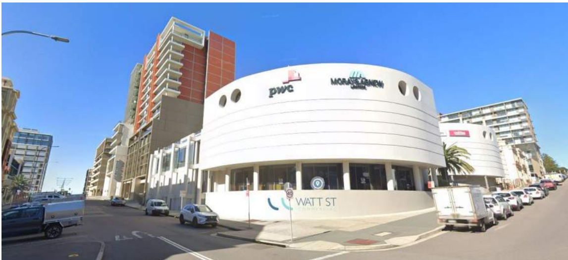
Figure 62: 45 Watt Street, Newcastle - corner of Watt and King streets facing east (Source: Google Streetview)
