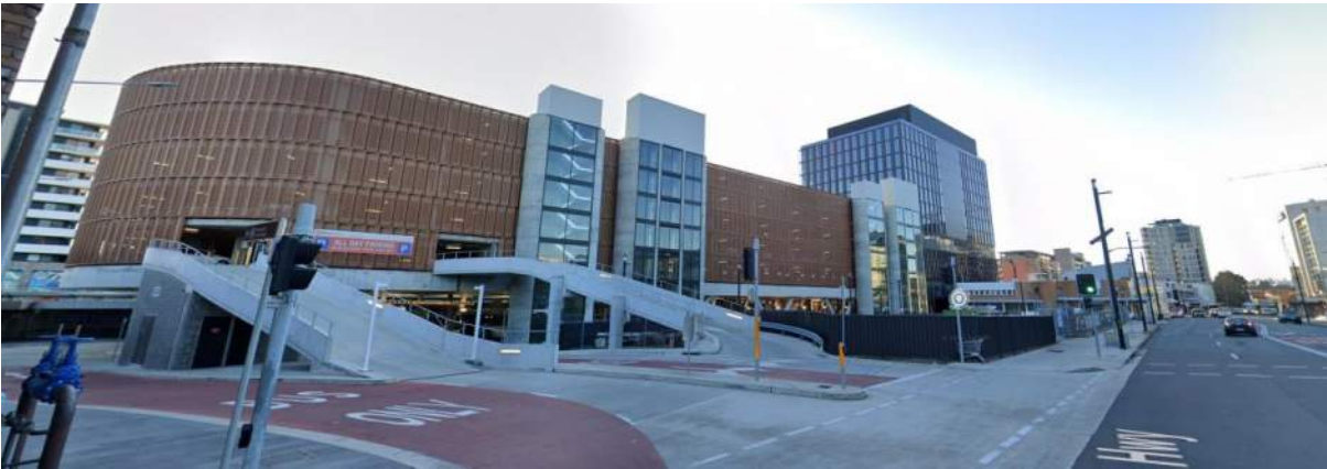
Figure 126: 874 Hunter Street, Newcastle West facing east (Source: Google Streetview)
