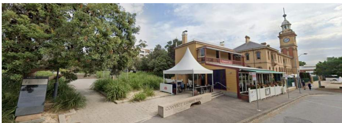
Figure 29: Convict Lumber Yard, Paymasters Cottage, and Newcastle Customs House, Newcastle East (Source: Google Streetview)
