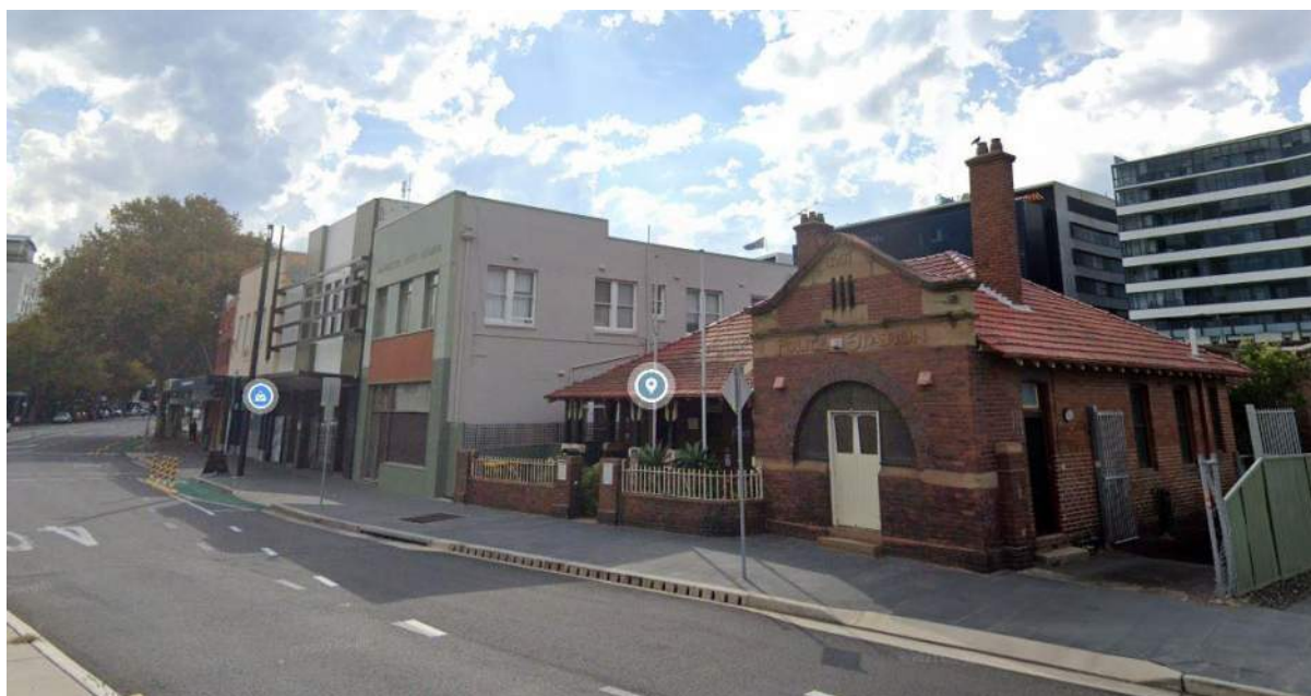
Figure 98: 558 Hunter Street, Newcastle facing west (Source: Google Streetview)
