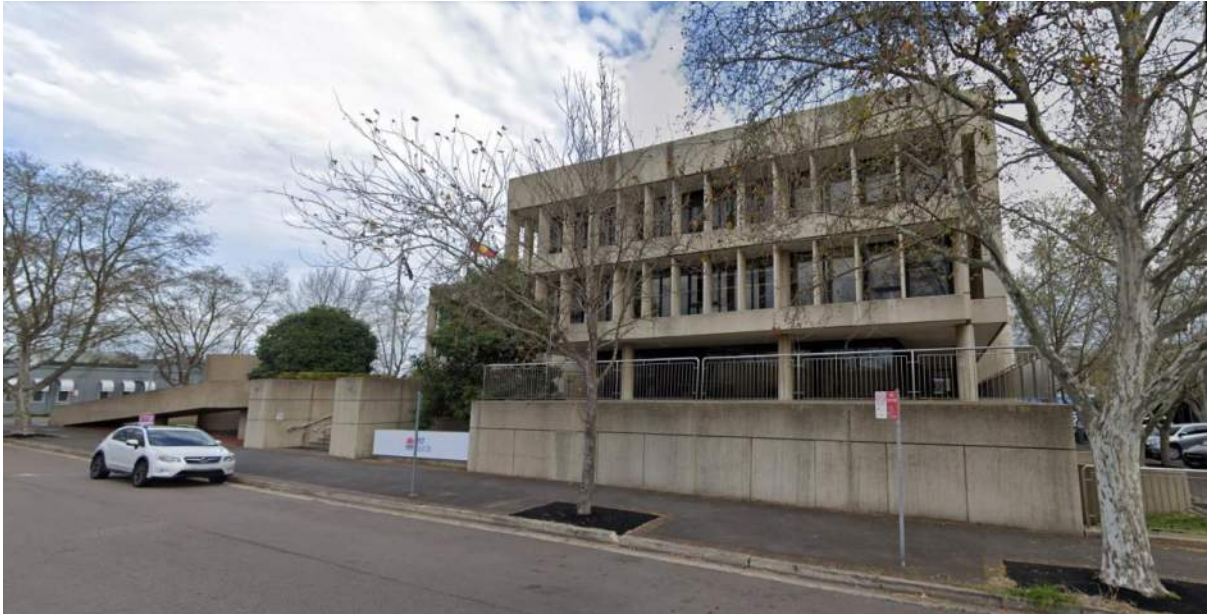
Figure 115: 117 Bull Street, Newcastle West (Source: Google Streetview)
