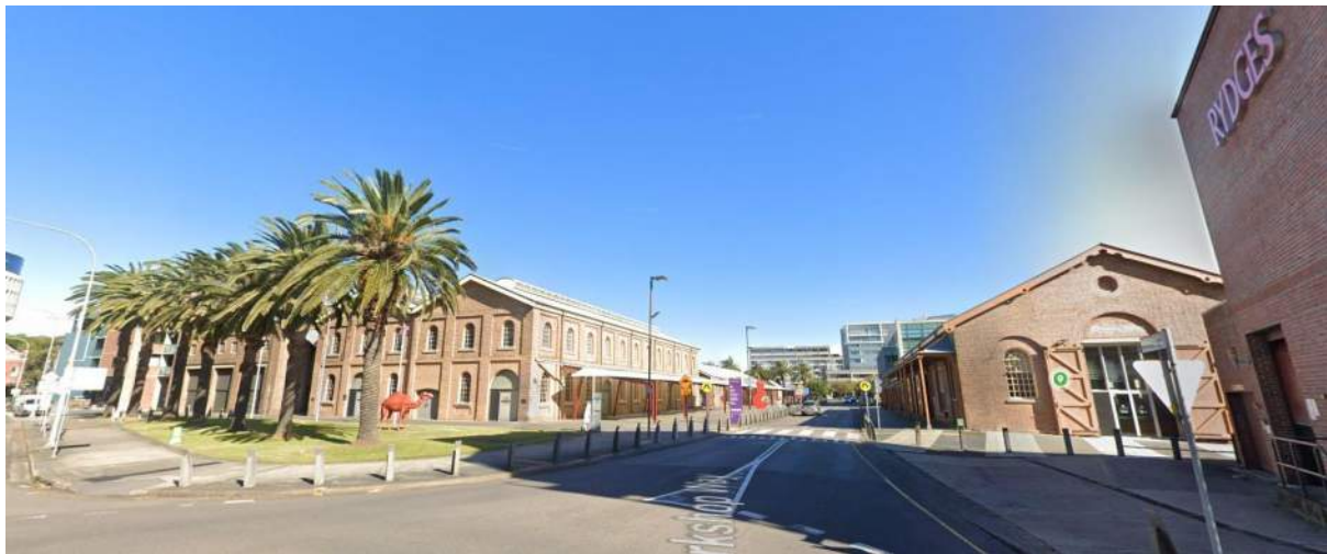
Figure 76: Civic Railway Workshops (Source: Google Streetview)
