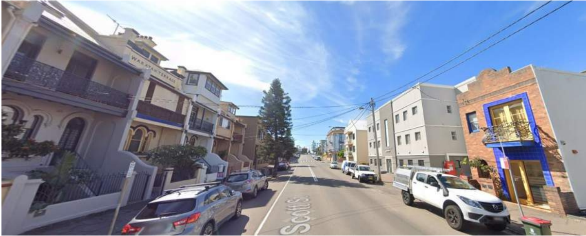
Figure 33: 52 and 33 Scott Street, Newcastle East facing east (Source: Google Streetview)
