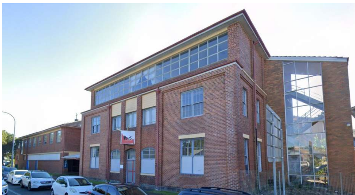
Figure 129: 246 Parry Street, Newcastle West (Source: Google Streetview)
