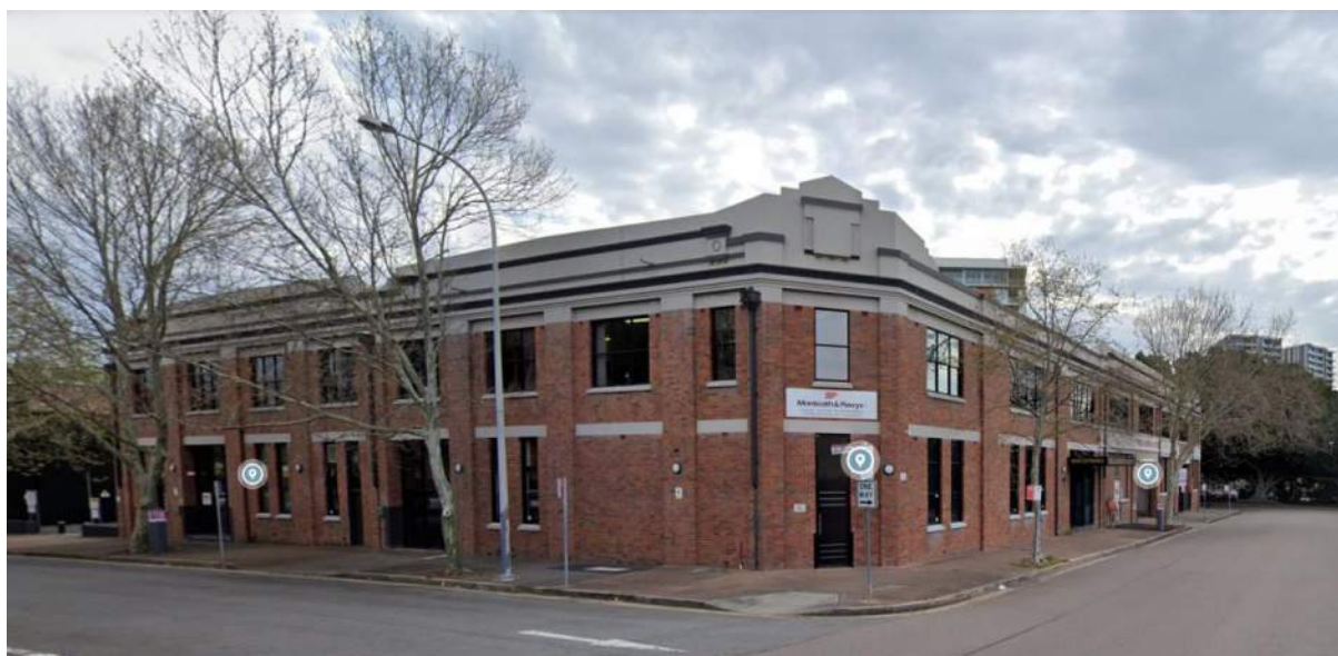
Figure 116: 125 Bull Street, Newcastle West (Source: Google Streetview)
