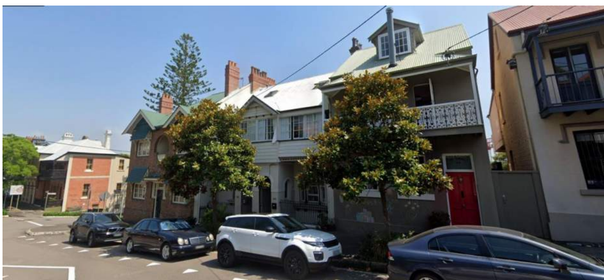
Figure 65: 58 Church Street, The Hill facing west (Source: Google Streetview)
