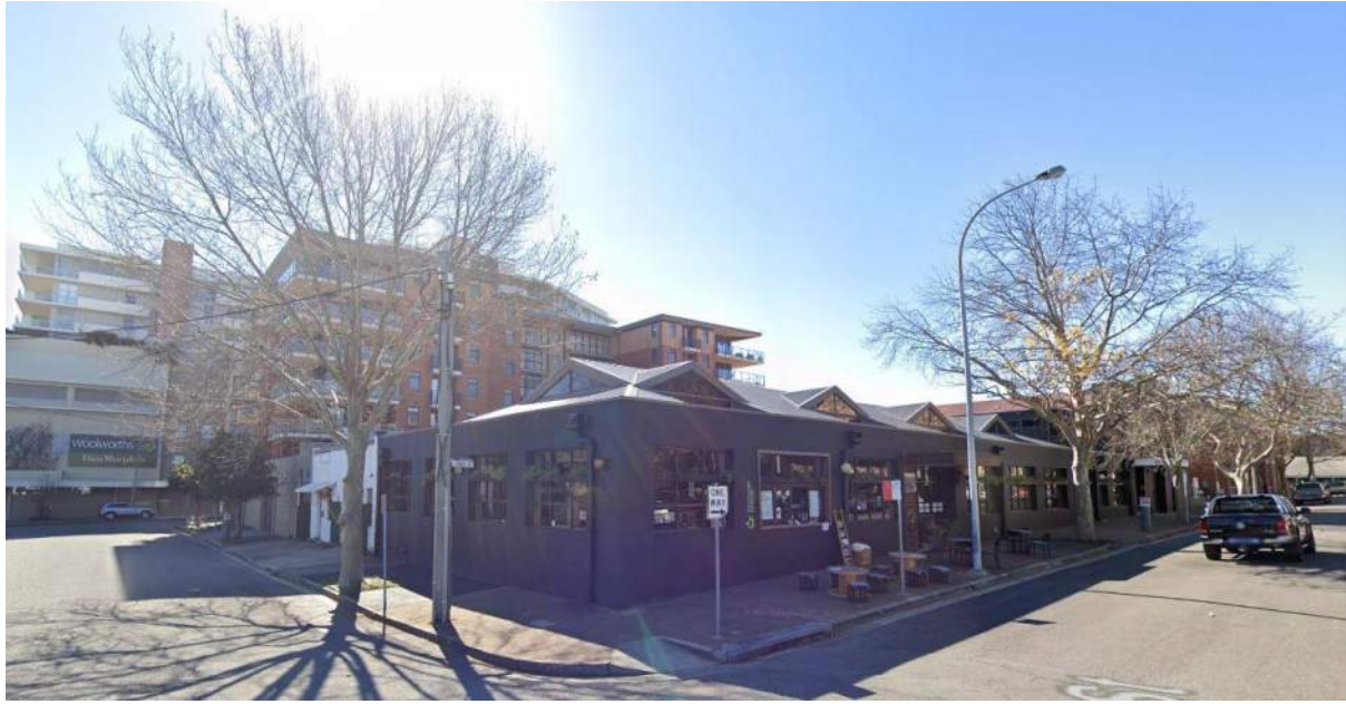
Figure 111: 6 Dick Street, Newcastle West facing north (Source: Google Streetview)
