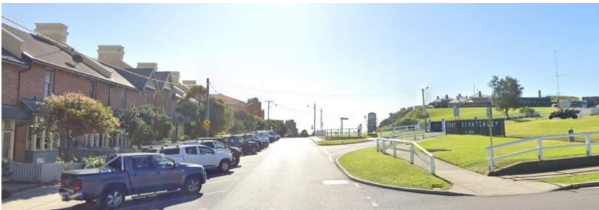
Figure 34: Boatman's Terrace Group and Fort Scratchley, Newcastle East facing north (Source: Google Streetview)
