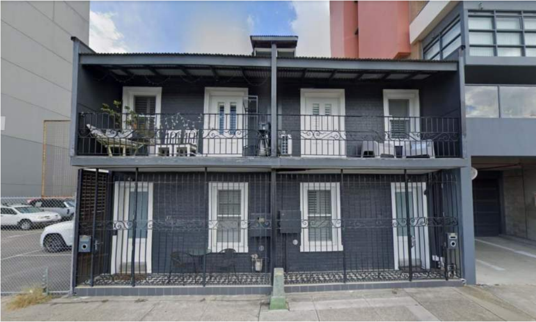
Figure 135: 17 and 19 Beresford Street, Newcastle West (Source: Google Streetview)
