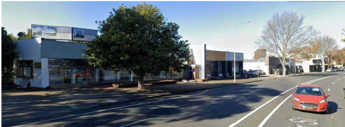
Figure 124: 990 Hunter Street, Newcastle West facing east (Source: Google Streetview)
