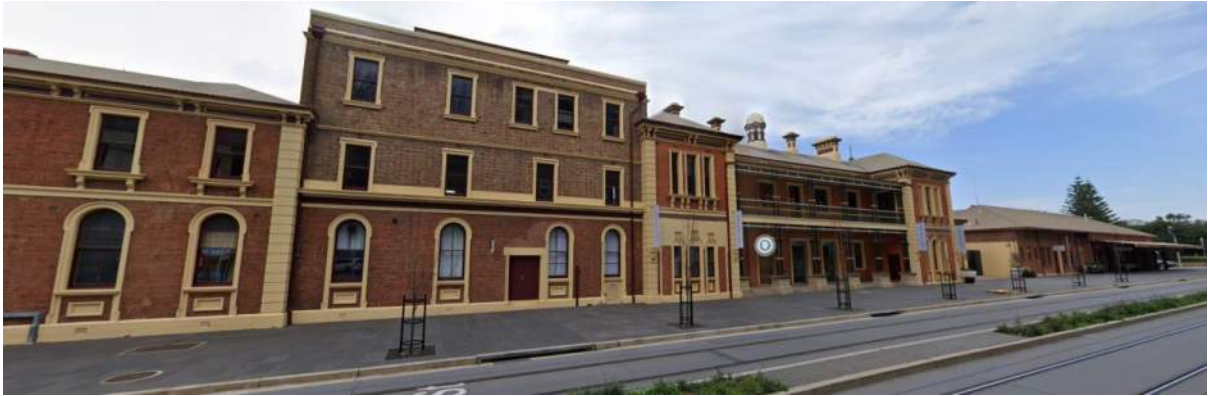
Figure 50: Newcastle Railway Station at 110 Scott Street, Newcastle (Source: Google Streetview)
