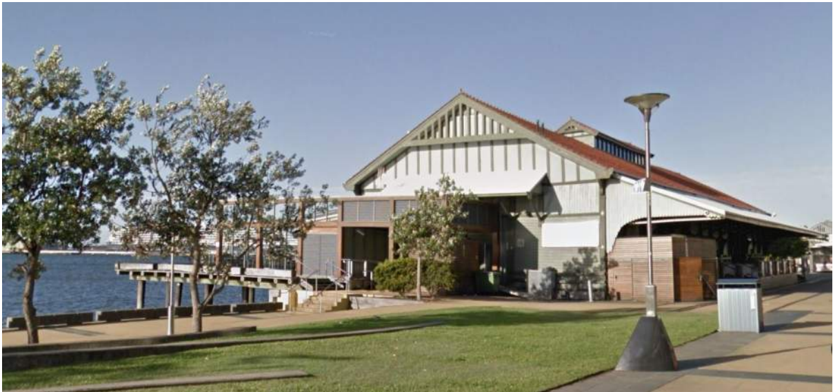
Figure 74: No.2 Lee Wharf - Building C (Source: Google Streetview)
