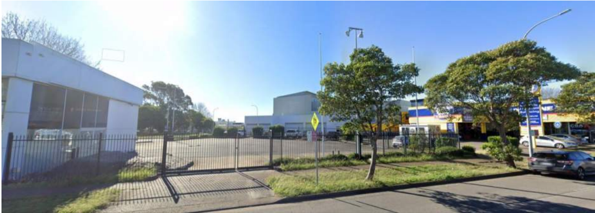
Figure 125: 214 Parry Street, Newcastle West facing north (Source: Google Streetview)
