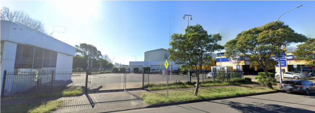
Figure 125: 214 Parry Street, Newcastle West facing north (Source: Google Streetview)
