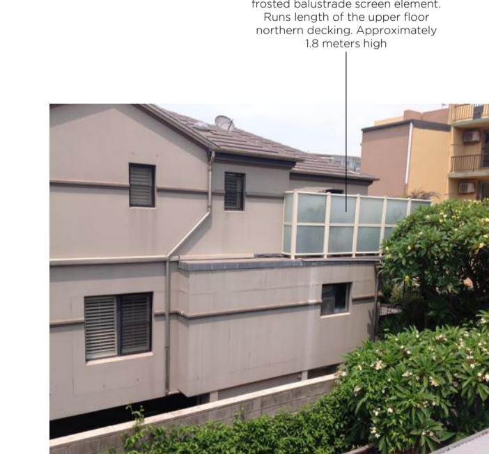
07. view south west
