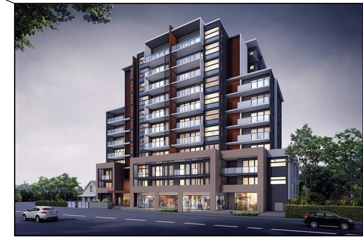
NEARBY DEVELOPMENT PROPOSAL CURRENTLY UNDER CONSTRUCTION
