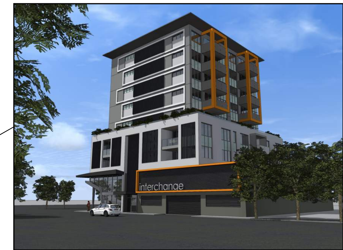
NEARBY DEVELOPMENT UNDER CONSTRUCTION
