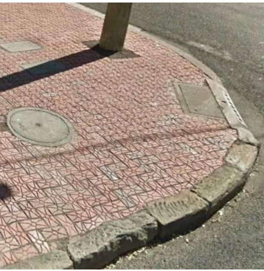
EXAMPLE OF PAVING BRICKS USED IN NEWCASTLE AND PARTICULARLY IN WICKHAM (SOURCE: GOOGLE STREET VIEW)
