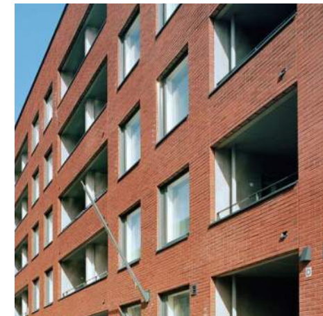
FACE BRICKWORK EXAMPLE
