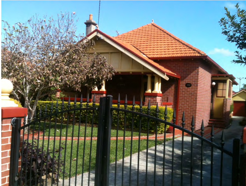
Figure 2.6 – A bungalow on Corlette Street. The dwelling contributes in a positive manner to the streetscape
