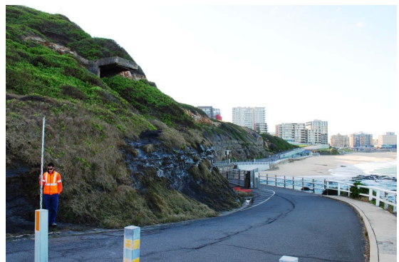
Geo-hazard #6 – Tension crack & settlement of coastal edge of Shortland Esplanade. Hazard associated with deep fill supported by an old mortar block retaining wall
