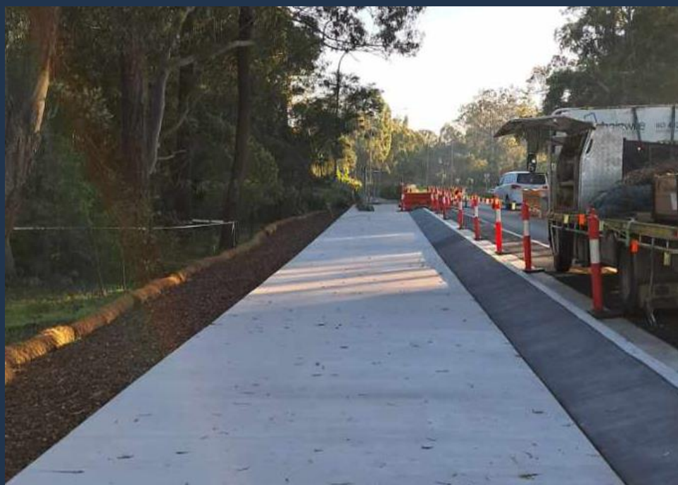
Underway: Construction of shared pathway at Minmi Road Fletcher.
