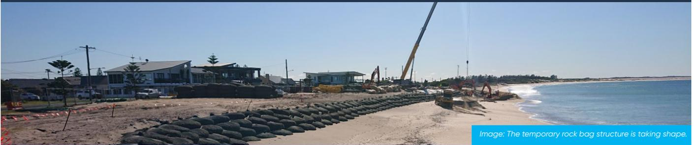
Image: The temporary rock bag structure is taking shape.
