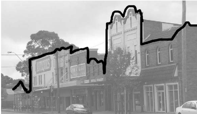
Figure 6: Existing parapets dominating the street edge
