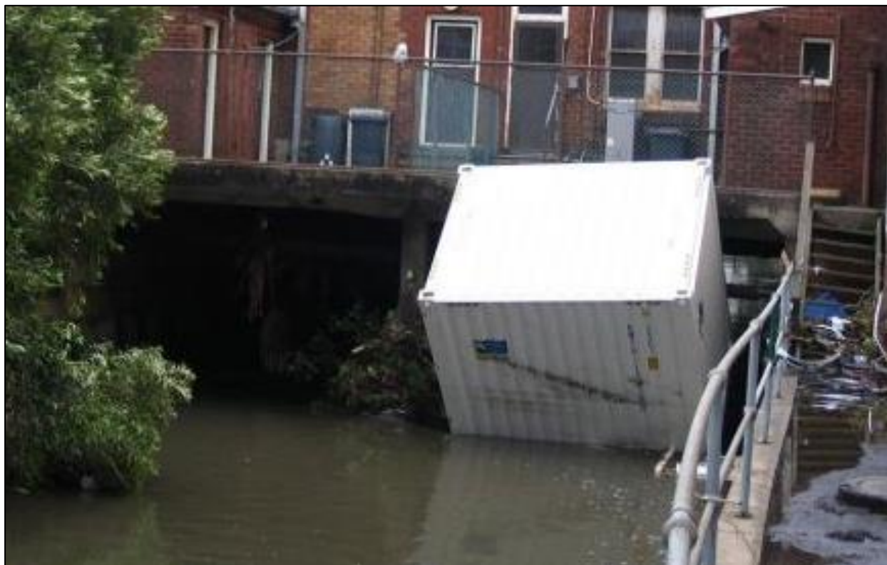
Plate 5 Photo taken following 2007 flood showing shipping container blocking culvert beneath 681 Hunter Street (BMT WBM, 2012)
