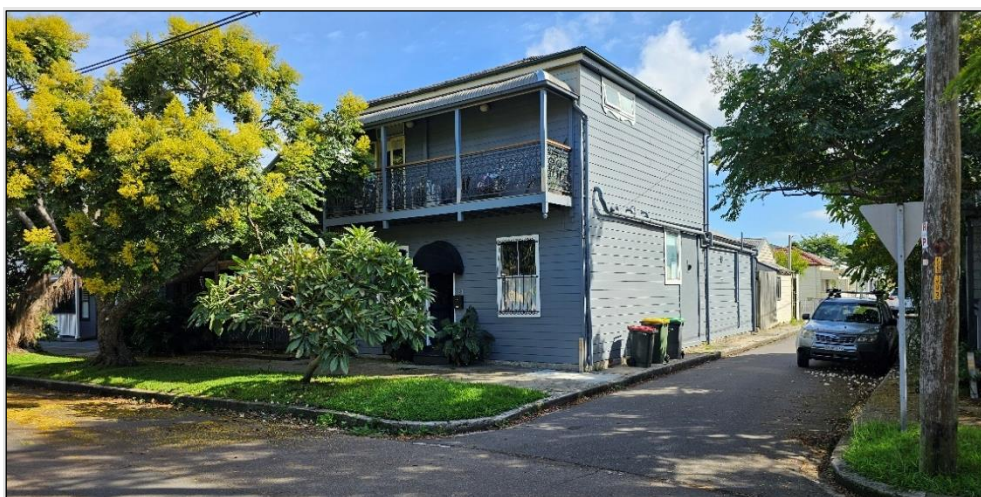
Figure 2 - Site frontage from Hargrave Street Carrington
