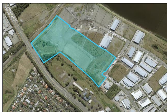
Figure 1: Subject Land - 60 Riverside Drive Mayfield West
