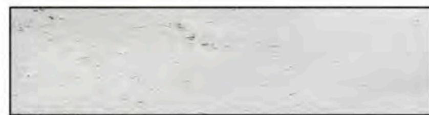
Off form Concrete
