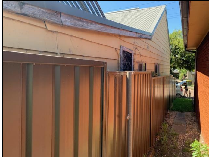
Figure 3: Windows on eastern elevation of 55 Henry Street
