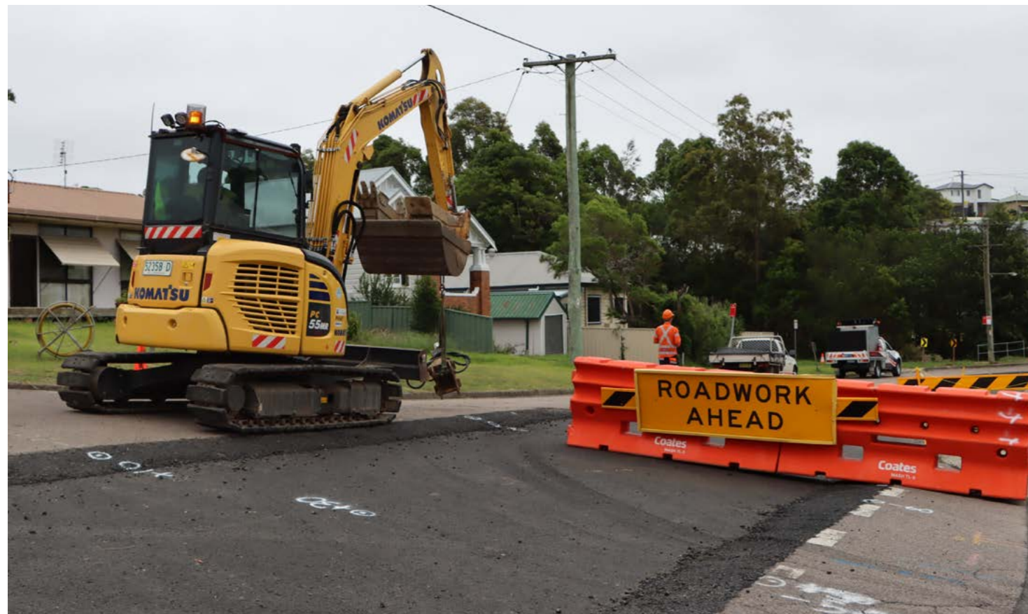
Work progressing on road reconstruction projects at Irrawang Street, Wallsend.
