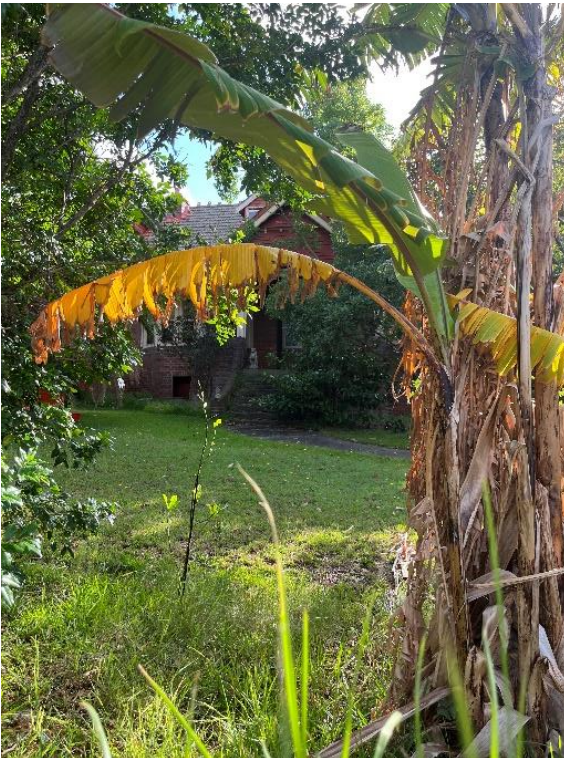
Figure 27: View from Regent Street across the front lawn
