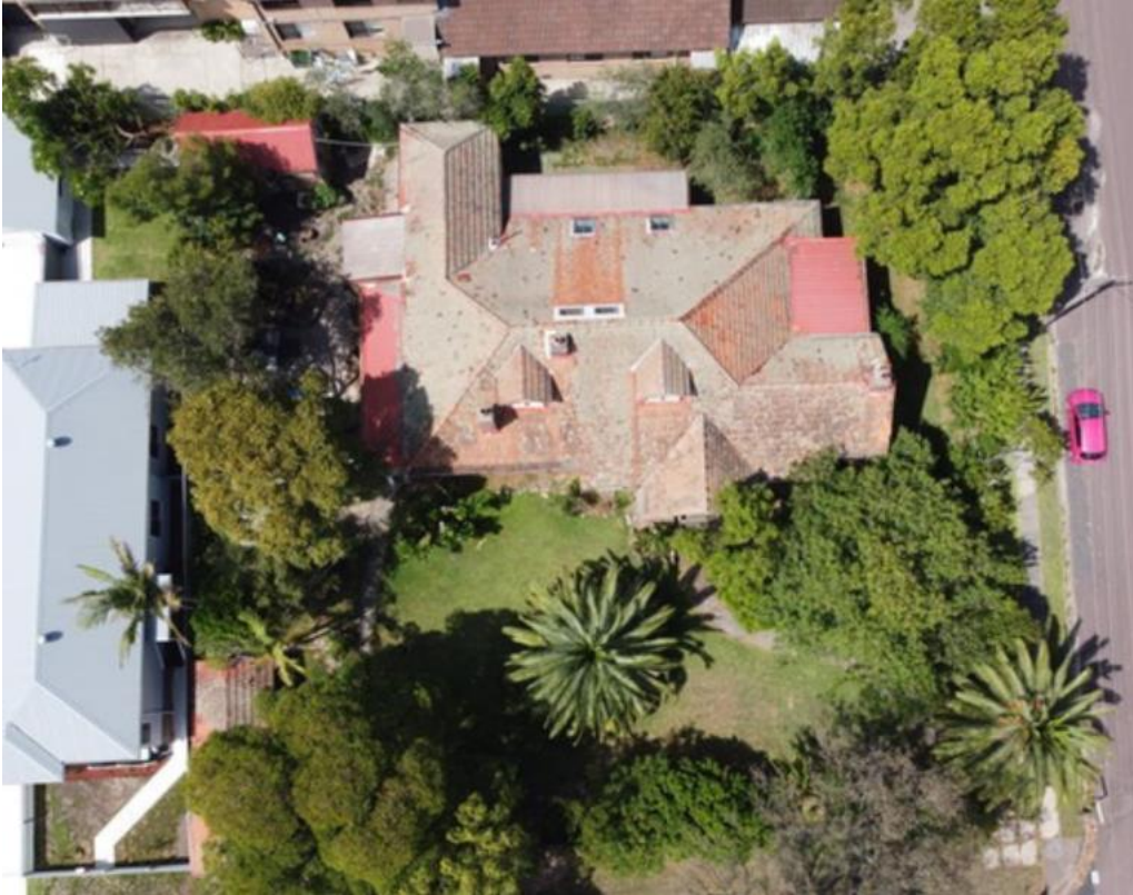
Figure 2: Aerial View of the site at 22 Victoria Street Mayfield https://www.domain.com.au/property-profile/22-victoria-street-mayfield-nsw-2304
