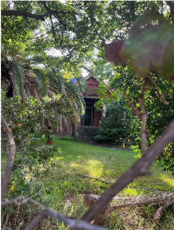
Figure 28: View from Regent Street across the front lawn to the entry porch
