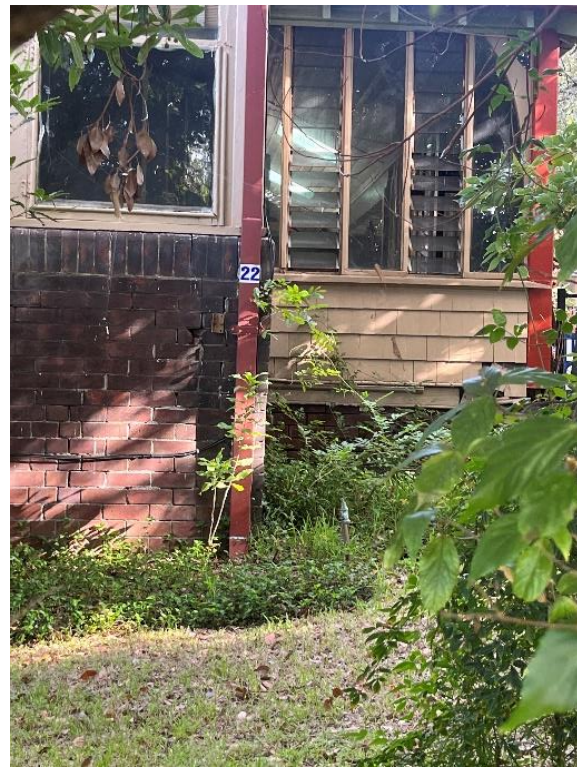
Figure 24: Rear enclosed verandah with timber shingled cladding and louvred windows.
