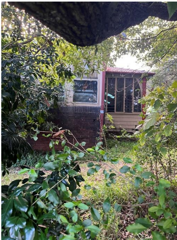
Figure 23: East elevation showing rear enclosed verandah
