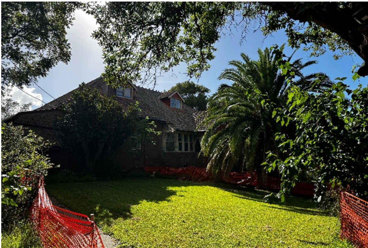
Figure 3 Southwestern elevation of 22 Victoria Street, Mayfield. (Source: CN, 2024)
