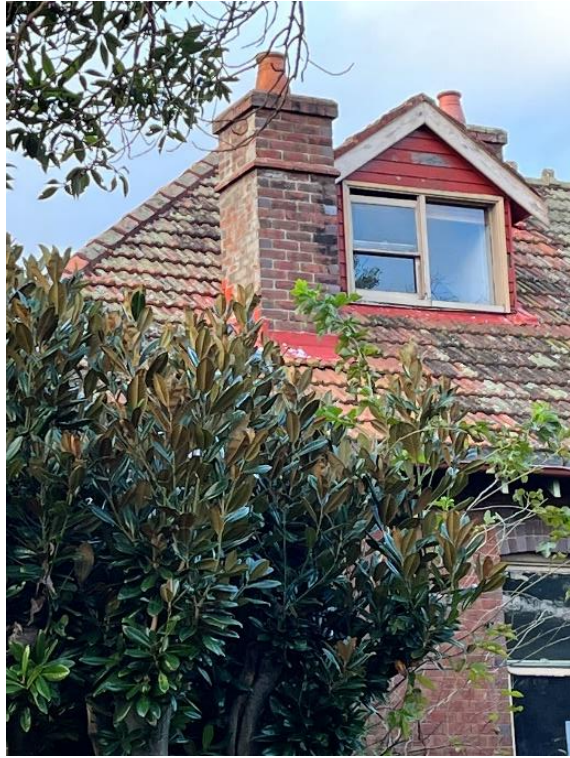
Figure 22: West side dormer
