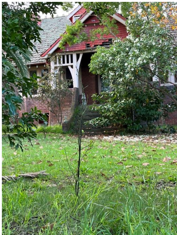
Figure 16: View of front entry from Regent Street
