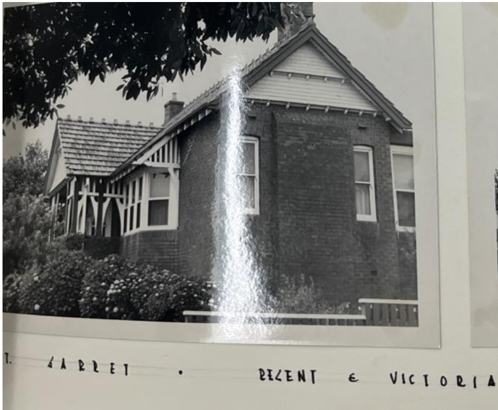
Figure 11: Photo of the east elevation of 22 Victoria Street Mayfield from Victoria Street, Mayfield. Date unknown. Source: "The Work of F.G. Castleden, 1907–1919: An Architectural Thesis" John Sara.
