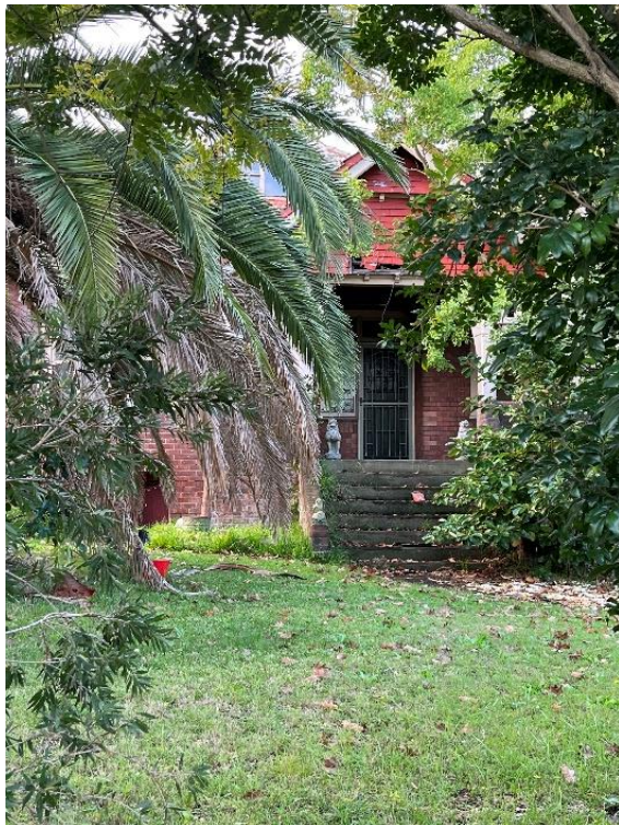
Figure 15: View of front entry from Regent Street
