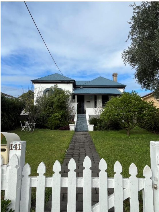
Figure 13: 141 Crebert Street, Mayfield
