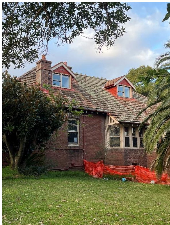
Figure 20: Later addition dormer windows
