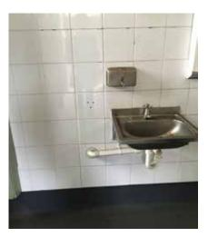
Figure 134: Basin with drainage through wall to the ladies WCs Source: TZG 2017
