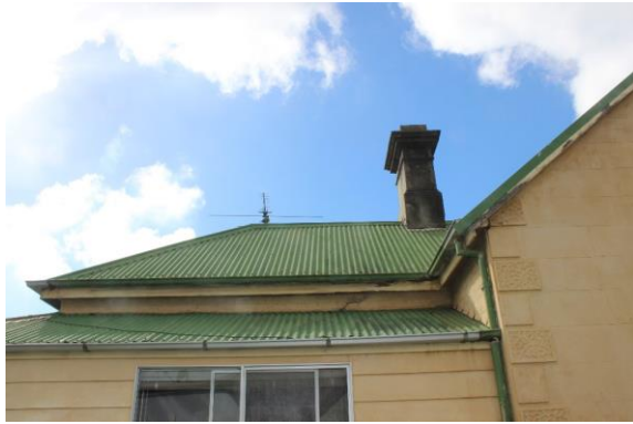
Figure 24: West elevation of enclosed verandah clad in Hardi plank boards.
