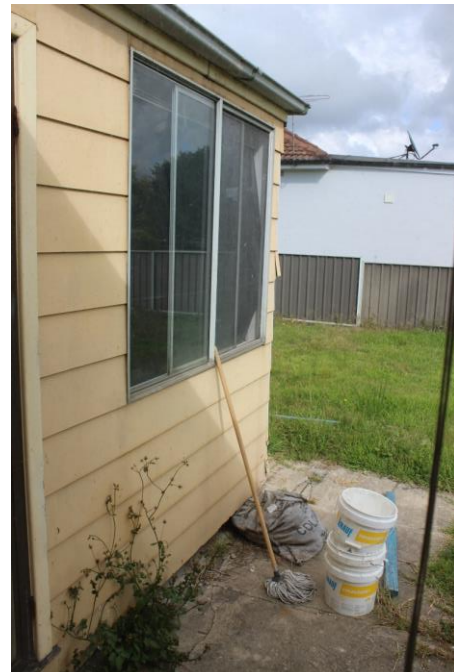
Figure 28: North elevation of rear addition clad in Hardi plank boards.
