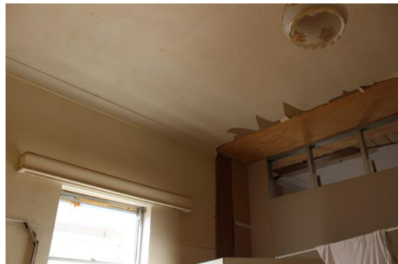
Figure 38: Partial removal of wall between the rooms.
