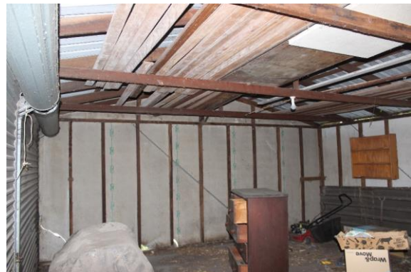
Figure 34: Interior of the fibro cement shed
