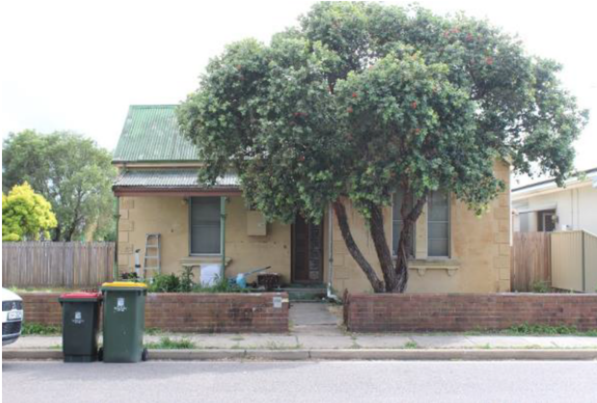
Figure 3 Street facing elevation of 14 Sunderland Street, Mayfield. (Source: Artefact, 2024)
