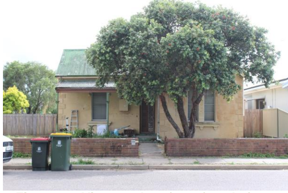
Figure 17; View north to front façade from Sunderland Street
