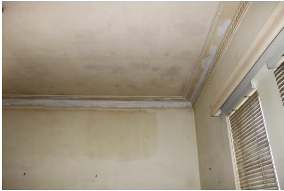
Figure 35: Interior ceiling of front room,
