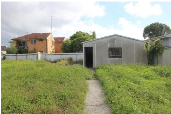
Figure 33: View north to the fibro cement clad shed at the rear of the site adjacent to the unnamed laneway.
