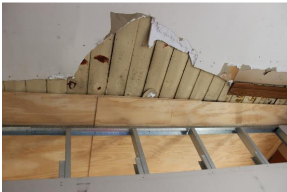
Figure 37: Original timber board ceiling is revealed under later hard plaster ceiling.
