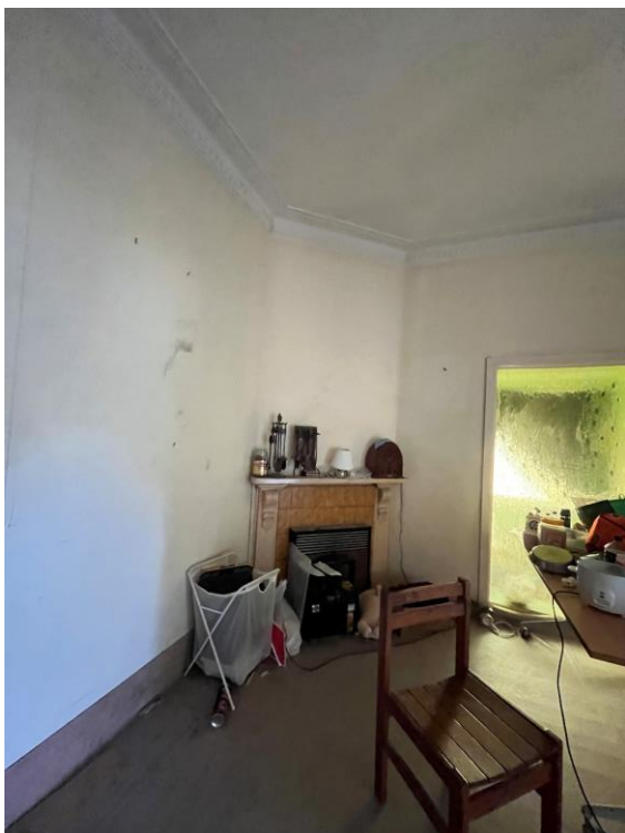
Figure 41: Remaining fireplace in the western back room.
