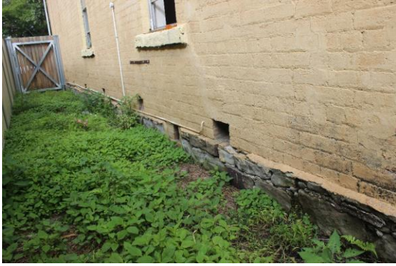
Figure 29: East elevation showing stone footing base under brick wall
