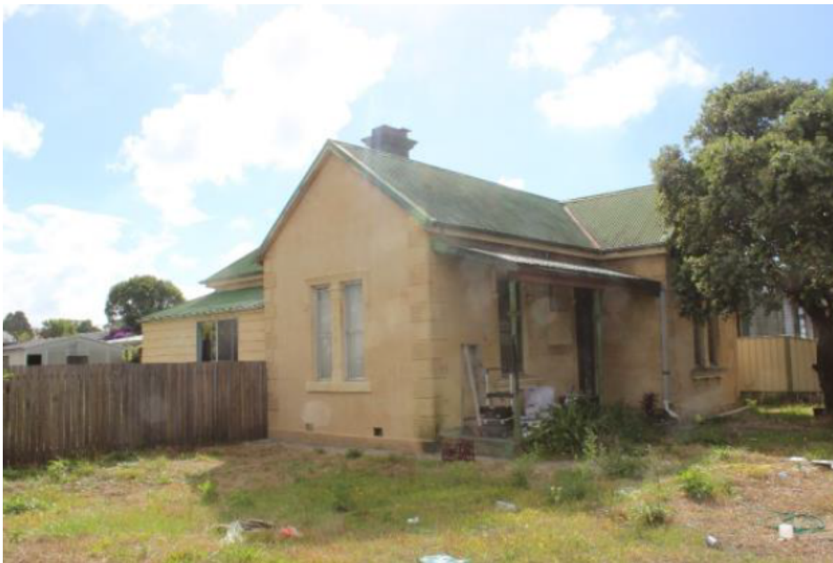
Figure 4 View of the property looking east from Sunderland Street. (Source: Artefact, 2024)
