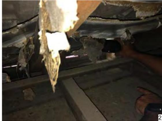
2. SHOWS TOP OF BRICKWORK ABOVE THIS SECTION OF EXTERNAL WALL. NO WALL PLATE IS PRESENT IN THIS SECTION AS IT IS IN OTHERS
