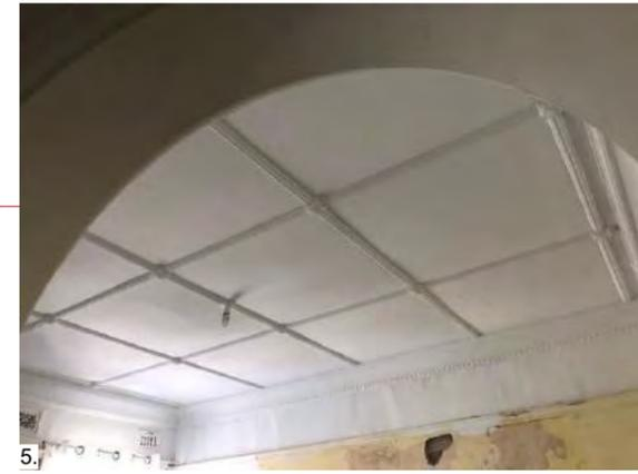
6. REPLACED CEILING WITHIN AFFECTED ROOM. PROVIDING EVIDENCE THAT THIS ROOM HAD BEEN DAMAGED AND REPAIRED IN THE PAST
