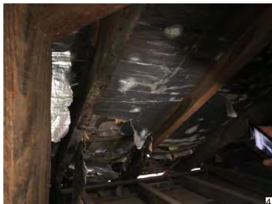
4. SHOWS MIXED TIMBER TYPES. THE DARKER TIMBER TO THE LEFT OF THE IMAGE IS OREGON AND APPEARS TO HAVE BEEN REUSED (UPSIDE DOWN) FROM PART OF THE ORIGINAL ROOF STRUCTURE.
