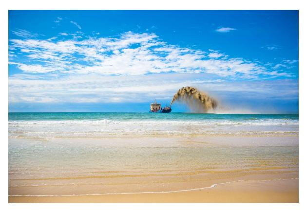
Figure 4: A TSHD rainbowing sand onto the nearshore area of the beach as part of beach nourishment works (source: City of Gold Coast).
