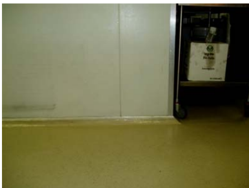
Picture 6: Epoxy coving on a coolroom floor
