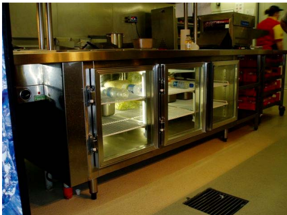
Picture 14 &15: Equipment elevated 150mm to permit cleaning underneath.
