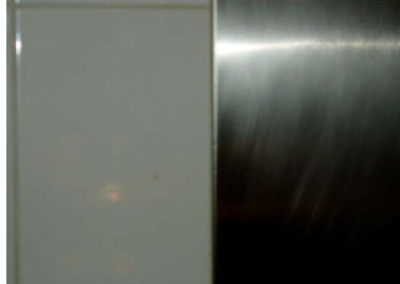
Picture 13: Stainless steel splashback sealed to a tiled wall surface.
