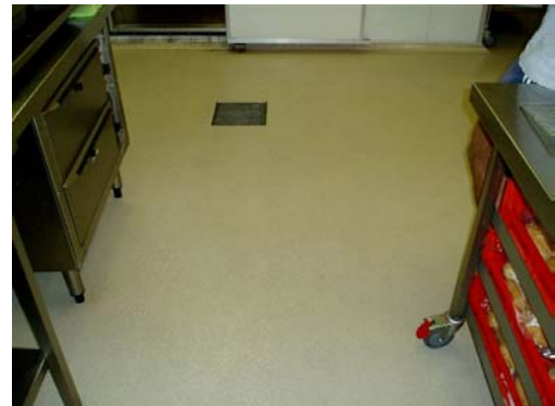
Picture 5: Floor waste
