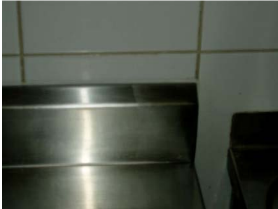
Picture 12: Sealing bench tops to wall.
