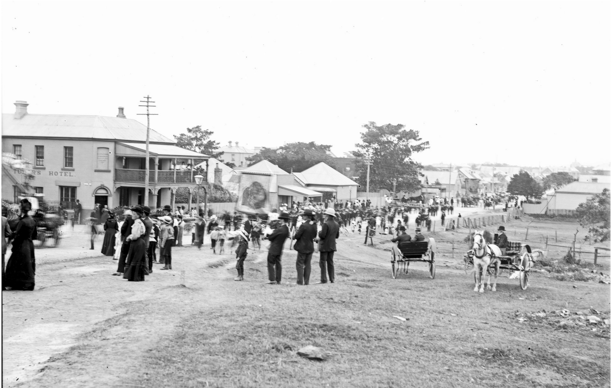
Figure 14: Denison Street, looking east, 28 October 1907. Tudor's Hotel, now the Hotel Bennett, is on the left. (Source: Ralph Snowball, 1907, held by Special Collections at the University of Newcastle, NSW)
