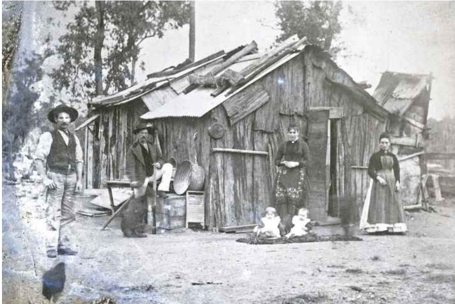
Figure 5: Typical Slab Hut, NSW (date unknown). (Source: Scanned from the original glass negative taken by Ralph Snowball. It is part of the Norm Barney Photographic Collection, held by Cultural Collections at the University of Newcastle, NSW, Australia)
