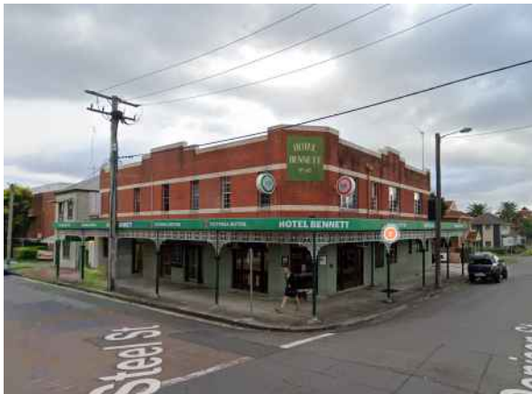
Figure 22: Hotel Bennett, corner of Denison and Steel Streets—LEP Item #124
