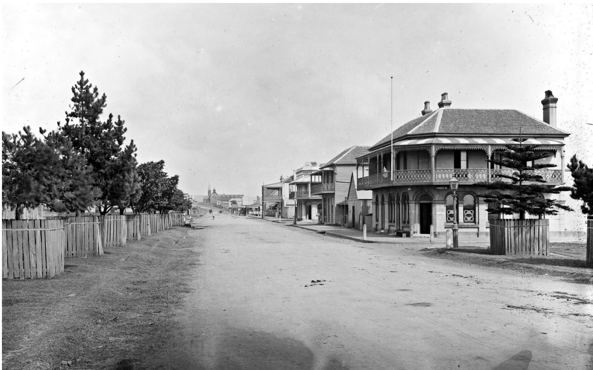
Figure 13: Denison Street, Hamilton (15 February 1892). The Universal Hotel can be seen in the foreground on the corner of Denison and Turner Streets. The former Hamilton Hotel, at 100 Denison Street, is visible beyond. St. Peter's Anglican Church is located in the background. (Source: Ralph Snowball, 1892, held by Special Collections at the University of Newcastle, NSW)
