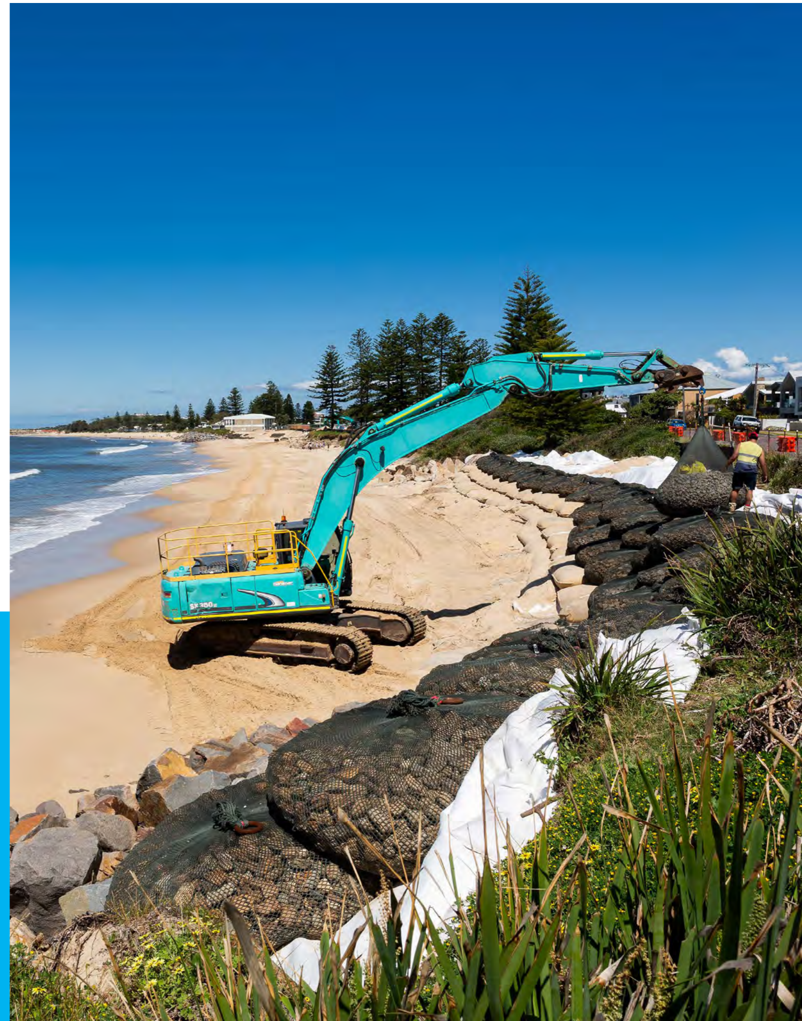
Works continue to protect Stockton's Coastline.
