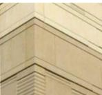
W2 PRECAST BANDED CONCRETE PANELS COL. SAND
