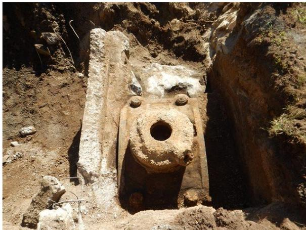
View to north showing concrete lined pit with a cast iron valve exposed in Foreshore Park Road in 2017. The valve is likely associated with the Zaara Street Power Station inlet and outlet water cooling channels.
