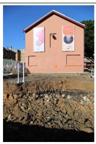
View to south showing excavation alongside Watt Street. Top of rubble reclamation fill exposed beneath compact gravel hard stand base.
