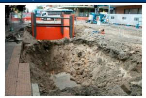
View to east towards Watt and Scott Street intersection showing sandstone rubble reclamation fill beneath Scott Street. Newcastle Station is immediately to left of photograph.
