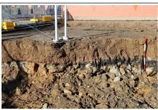
View to south showing excavation alongside Watt Street. Top of rubble reclamation fill exposed beneath compact gravel hard stand base.
