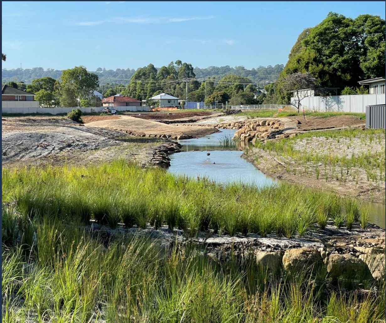
Image: Ironbark Creek Stage 5B Works
