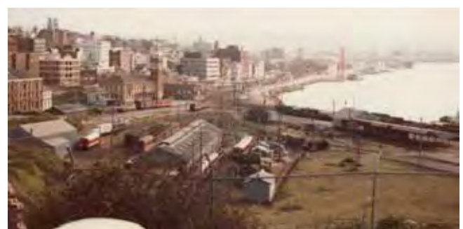
Photo from Fort Scratchley overlooking the Newcastle East Marshalling Yard in 1982 (source: www.railpage.com)
