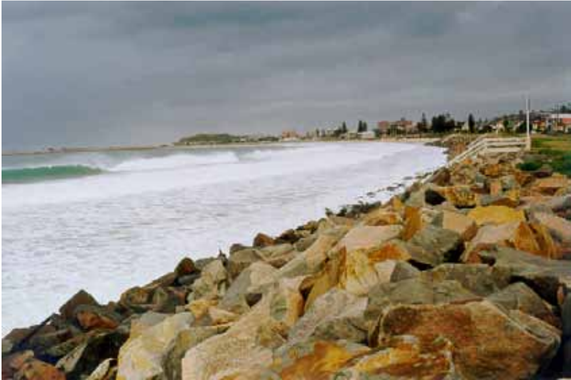
Plate 3 Mitchell Street seawall at Stockton Beach looking south. Part of the Newcastle skyline is in the background. (Source: WBM Oceanics Australia)
