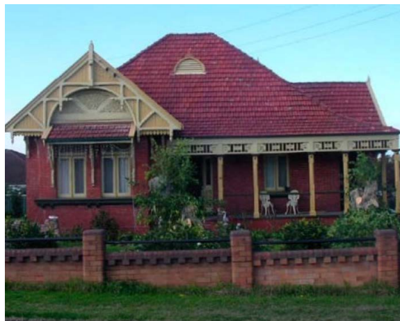
Figure 12: Example of an Edwardian house, Coomes Consulting (2006)
