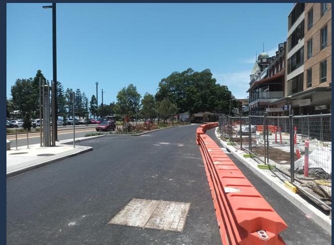
Underway: Stage 9 public domain works East End Newcastle.
