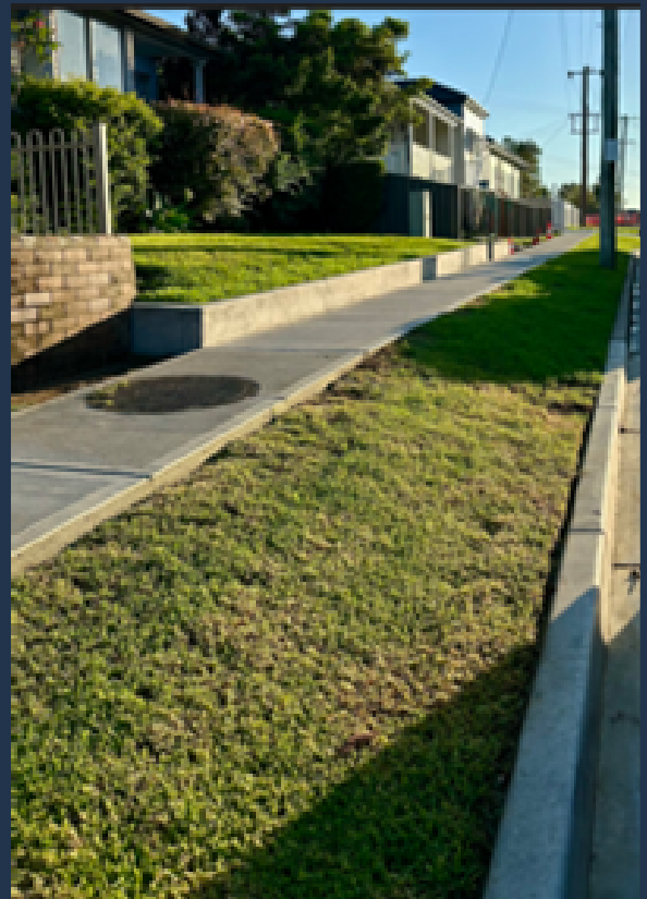
Underway: Traise Street Waratah.
