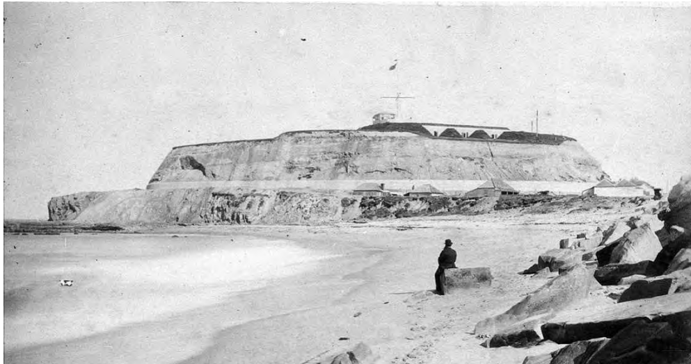
Figure 3.13. This view of Fort Scratchley in c1885, taken from the pier to Nobbys Head, shows the imposing concrete walls of the fortification, the casemates and the extant signal station (H B Ballard, Newcastle c1885, State Library of NSW, At World and Play BCP 05281)
