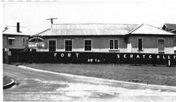
Figure 3.31. The former Ambulance station near the driveway entrance. Master Gunners Cottage at rear, circa 1965
