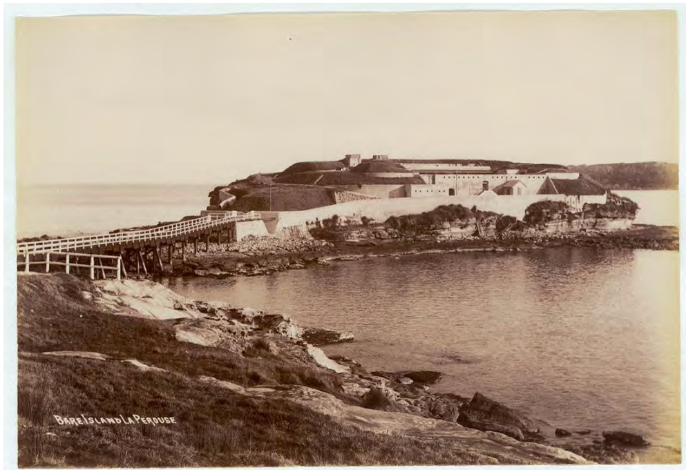
Figure 3.14. Bare Island Fort at La Perouse was built at the same time as Fort Scratchley, and was designed and executed by the same team of Jervois, Scratchley, Morrell and Barnet; similarly to Fort Scratchley, Bare Island Fort was an enclosed fortification constructed with massed concrete (Bare Island, La Perouse, c1900-10, State Library of NSW, PXE 711/177)
