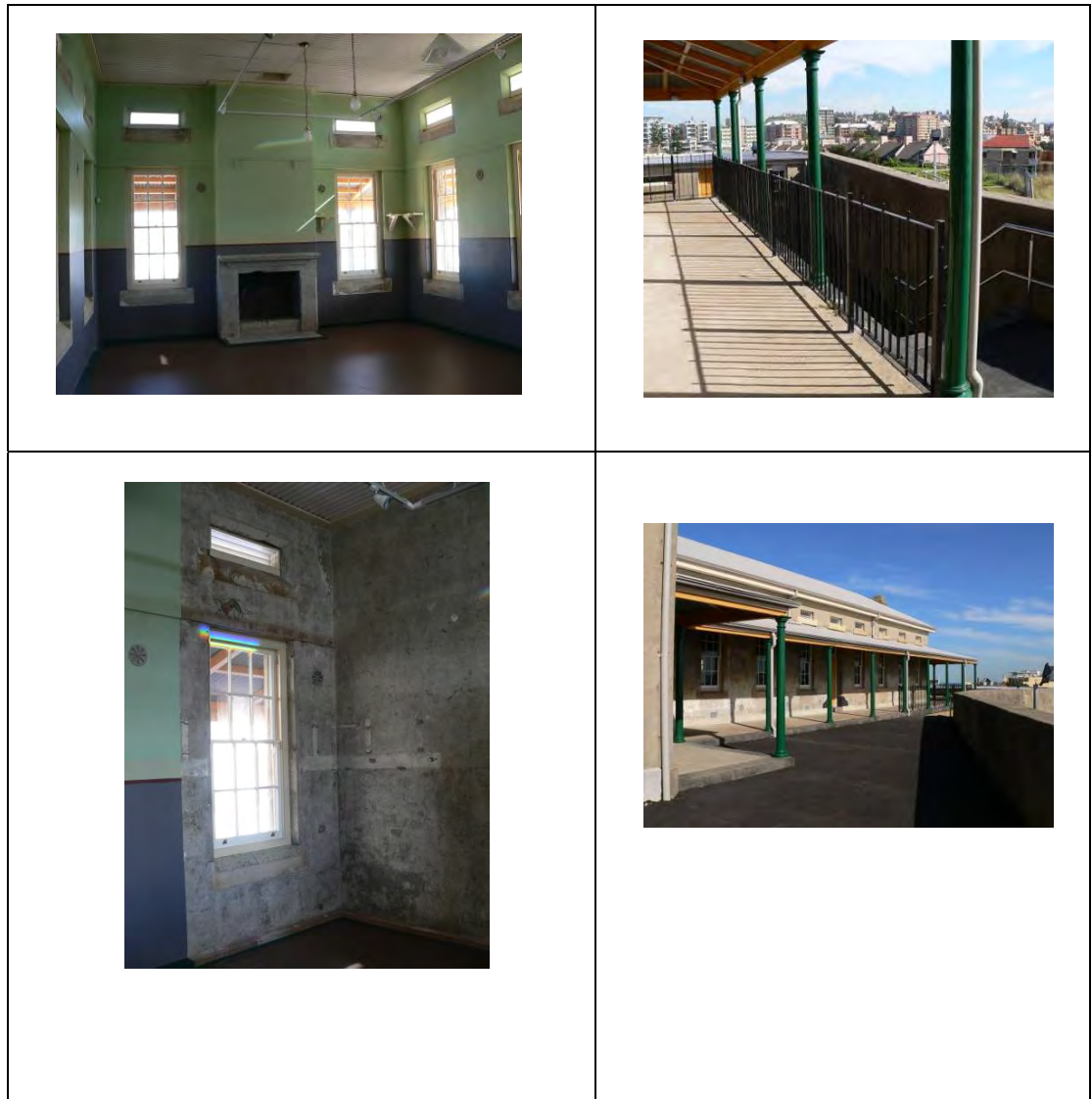
Figure 4.18 Barracks Building group - Barracks B21
