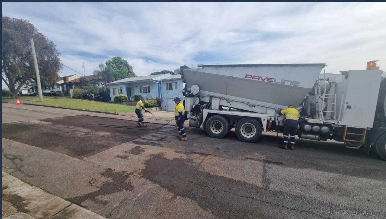
Coming up: Road resurfacing various locations City Wide
