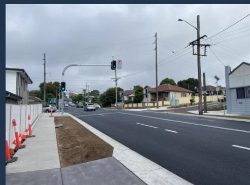
Underway: Construction of traffic control signals at Maud Street Waratah .
