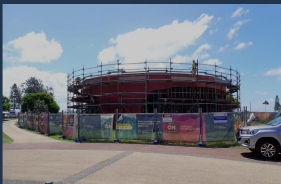
Underway: Construction of kiosk and amenities at Foreshore Park Newcastle East .
