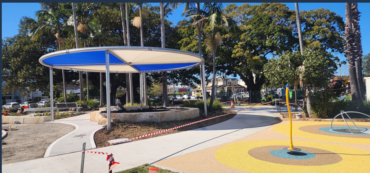
Underway: Amenities and playground construction at Gregson Park Hamilton.
