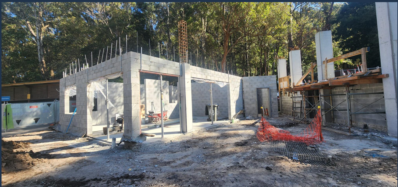
Underway: Construction of multi-purpose community facility at Blackbutt Reserve New Lambton.
