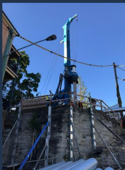
Image: Perkins Street Retaining Wall
