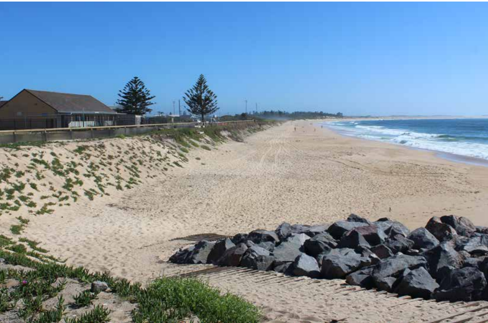
Figure 6. Northern section of Stockton Beach from northern end of Mitchell Street seawall. Former North Stockton Surf Life Saving Club building on back dune area now removed. (Photograph: MManning, CN, 4/1/19).
