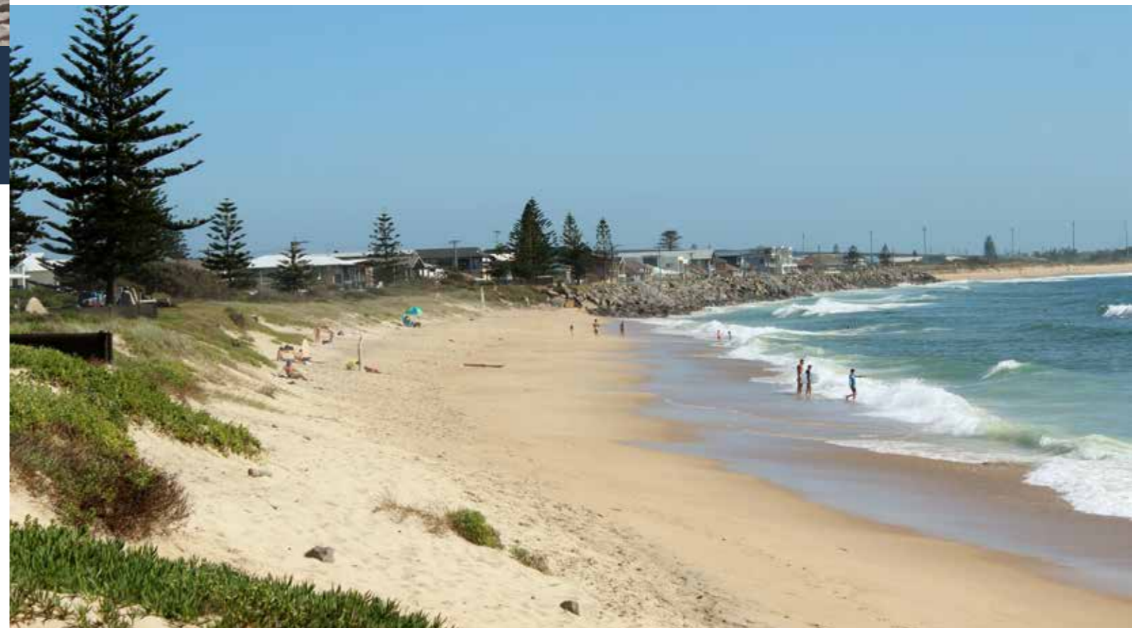
Figure 8. Central section of Stockton Beach with Mitchell Street seawall in midground (Photograph: MManning, CN, 4/1/19)
