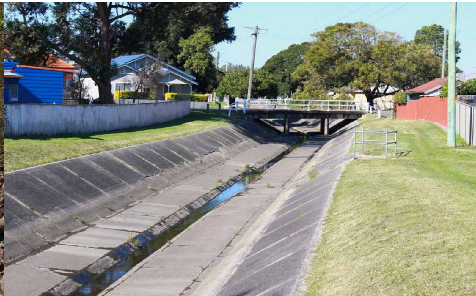
Figure 43. Throsby Creek (stormwater channel) looking east from Nile Street, Mayfield. (Photograph: MManning, CN, 21/7/19).
