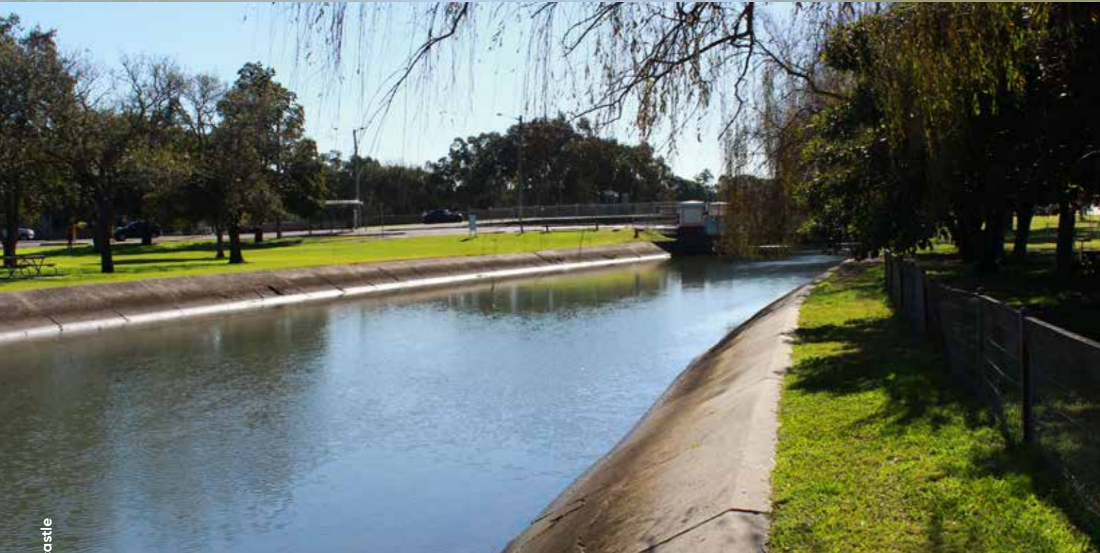
Figure 39. Throsby Creek (stormwater channel) entering tidal section of Throsby Creek near Maitland Road, Islington. (Photograph: MManning, CN, 21/7/19).
