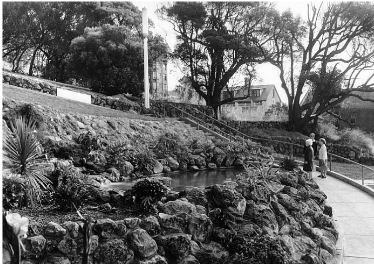
Figure 10 - The new rockeries and retaining walls, 1972.
