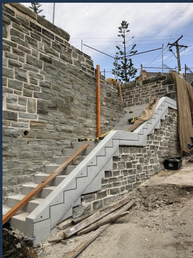
Retaining wall Perkins Street Newcastle
