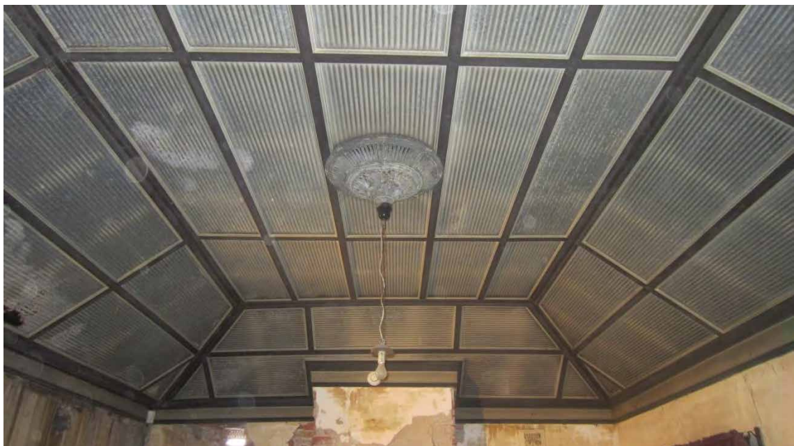
Figure 98. Dining room ceiling, showing ceiling rose for original gasolier (pre-electric lighting).
