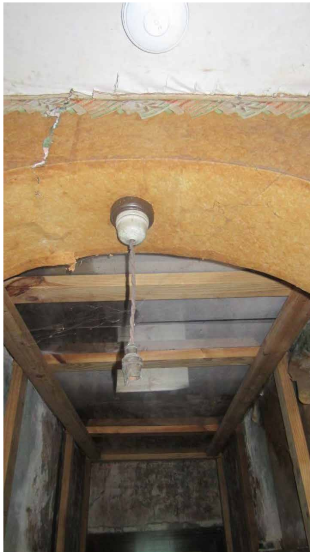
Figure 131. Hallway ceiling, west of archway; softwood and Perspex sheeting retain fretting plaster.
