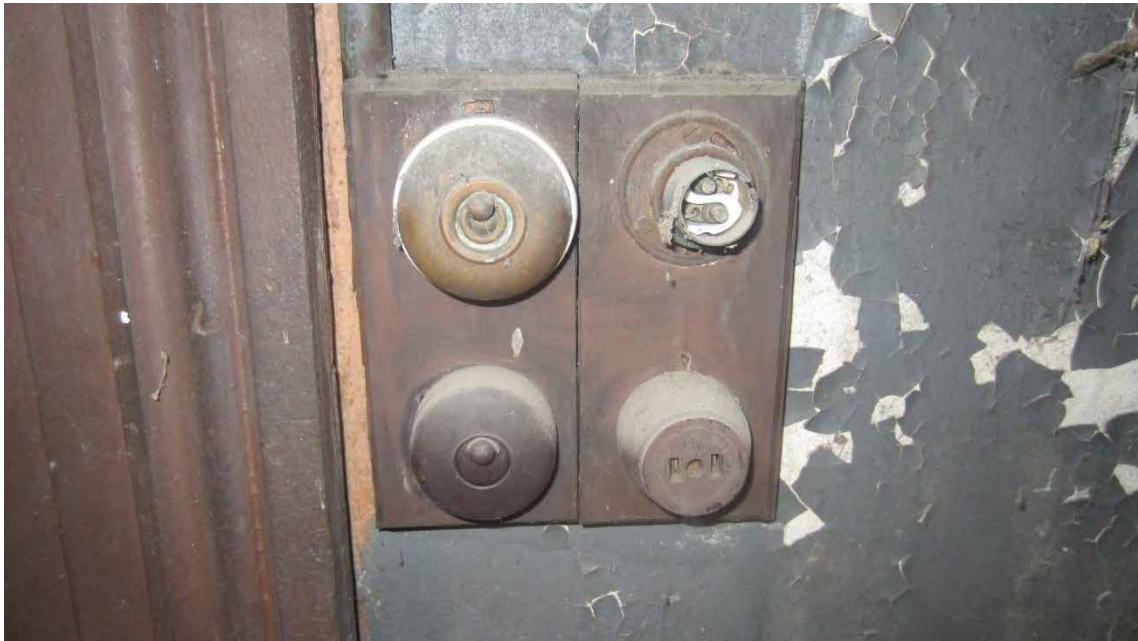
Figure 83. Early electric switches in kitchen, the oldest (brass) being for the bayonet light fitting, the lower (bakelite) with two-hole power point.
