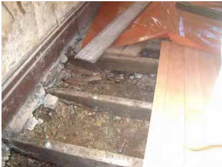
Figure 47. Relaying of floorboards. NSW Heritage Division
