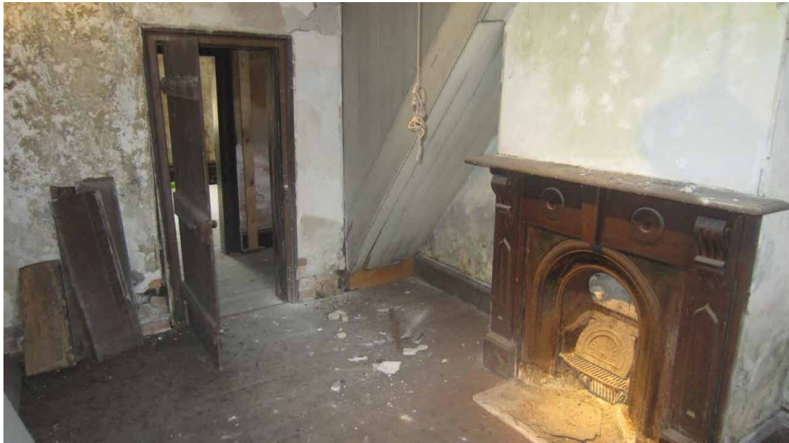
Figure 104. South-western bedroom; stairs lead to attic room. Note rustic finish of rear face of door leaf, contrasting with the much batter-finished other side addressing hallway.
