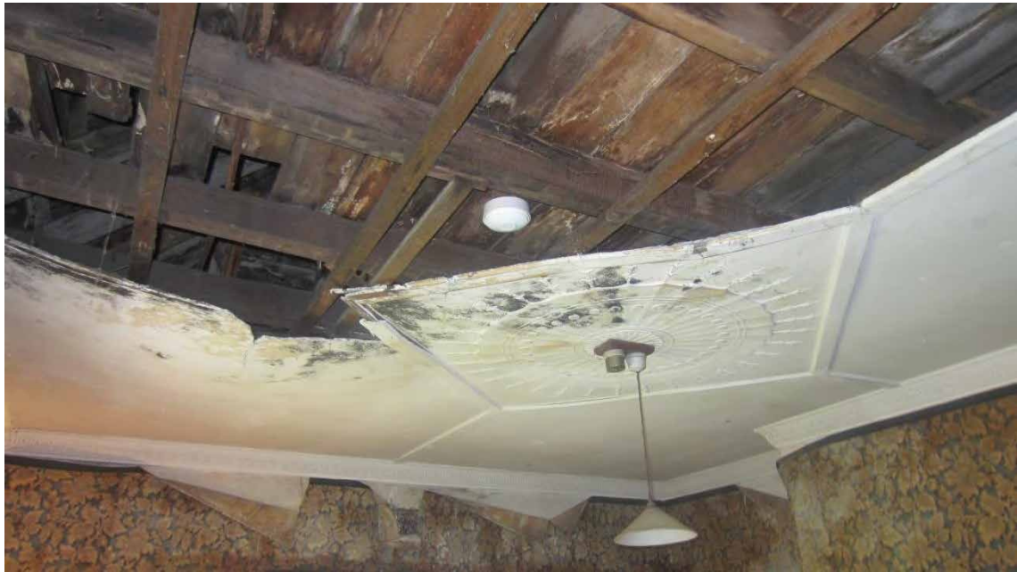
Figure 120. Damaged and depleted ceiling of south-eastern room (once also used at need as an office); ceiling dates from c. 1930s; nothing remains of original tongue in groove ceiling. Attic floor is visible.
