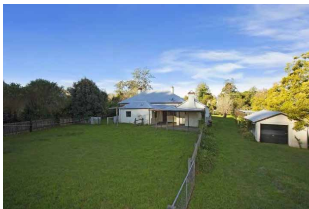
Figure 69. Rear elevation, showing kitchen on central axis, together with later side additions. McElwaine Property
