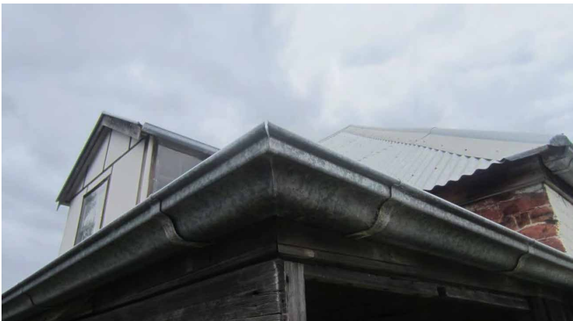
Figure 179. Unsoldered corner gutter join.
