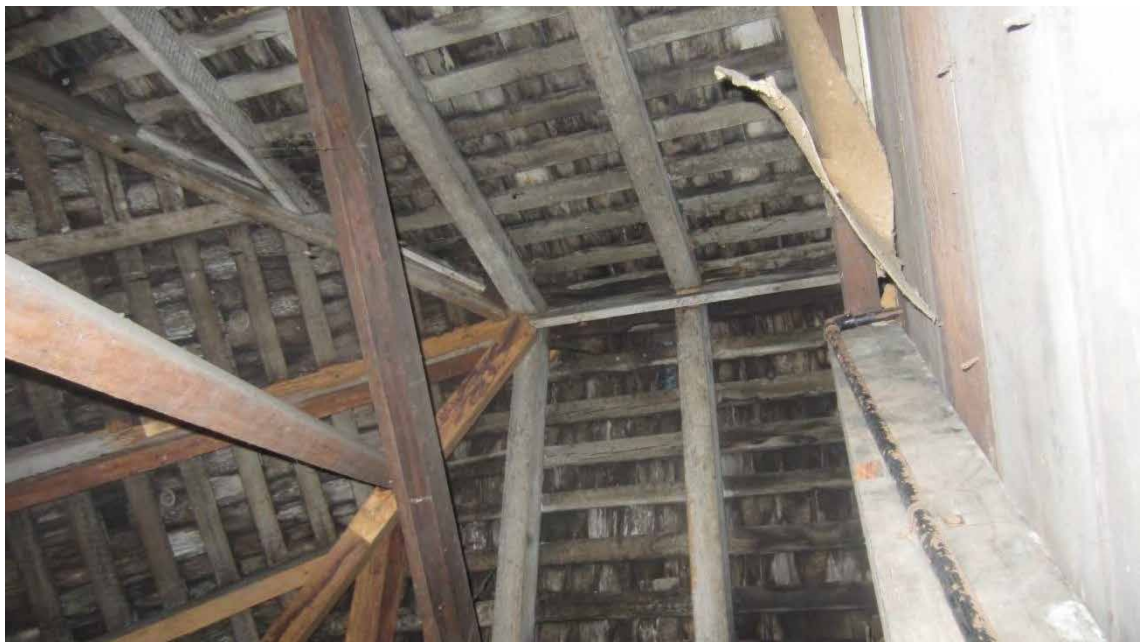
Figure 140. Battens support shingles externally concealed by galvanised iron.
