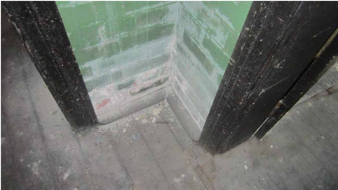
Figure 93. Damp damage at skirting level.
