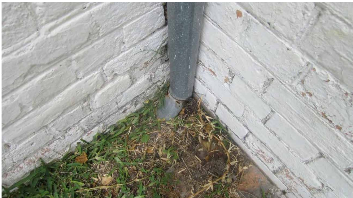
Figure 177. Downpipe not properly flashed into drain, leading to water penetration of walls.
