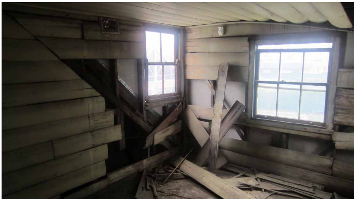
Figure 142. Dislocated lining boards.
