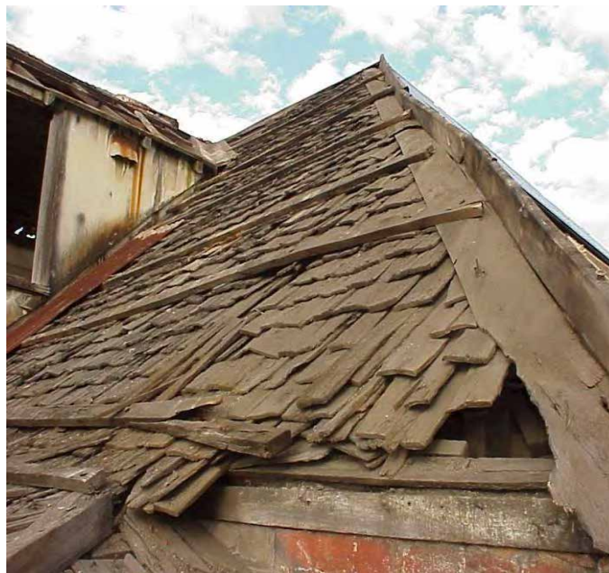
Figure 38. Shingle roof and dormer before conservation works. Suters Architects
