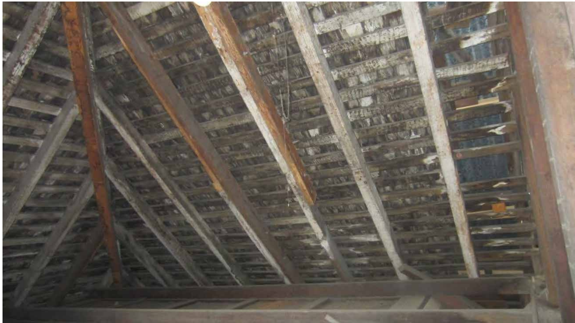
Figure 139. Roof cavity above dining room; new hardwood has been cleated to rafters following historic termite damage.
