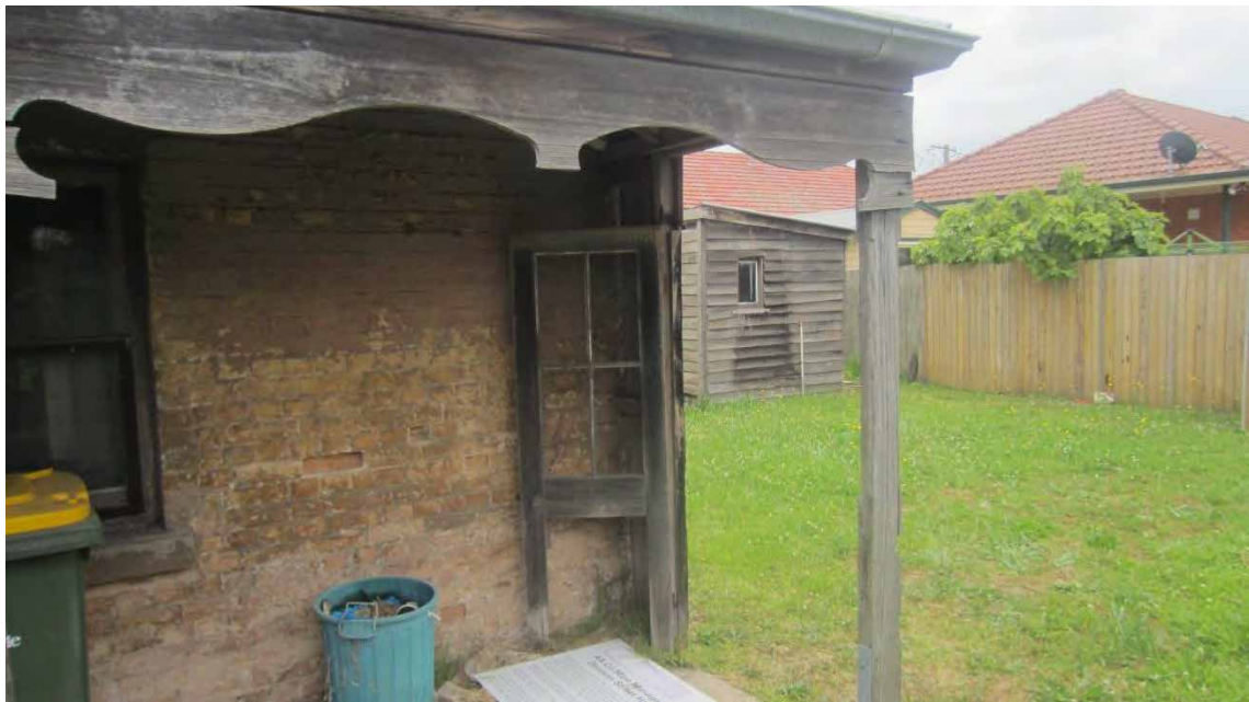
Figure 172. The missing panel of the door leaf formerly included a hatch allowing a ladder, for decades stored on the verandah and used for maintenance purposes, to be easily withdrawn when the door was closed.
