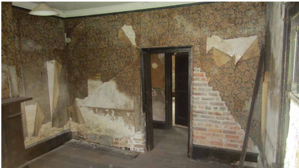
Figure 125. Note dislocated skirting board and peeling wallpaper.
