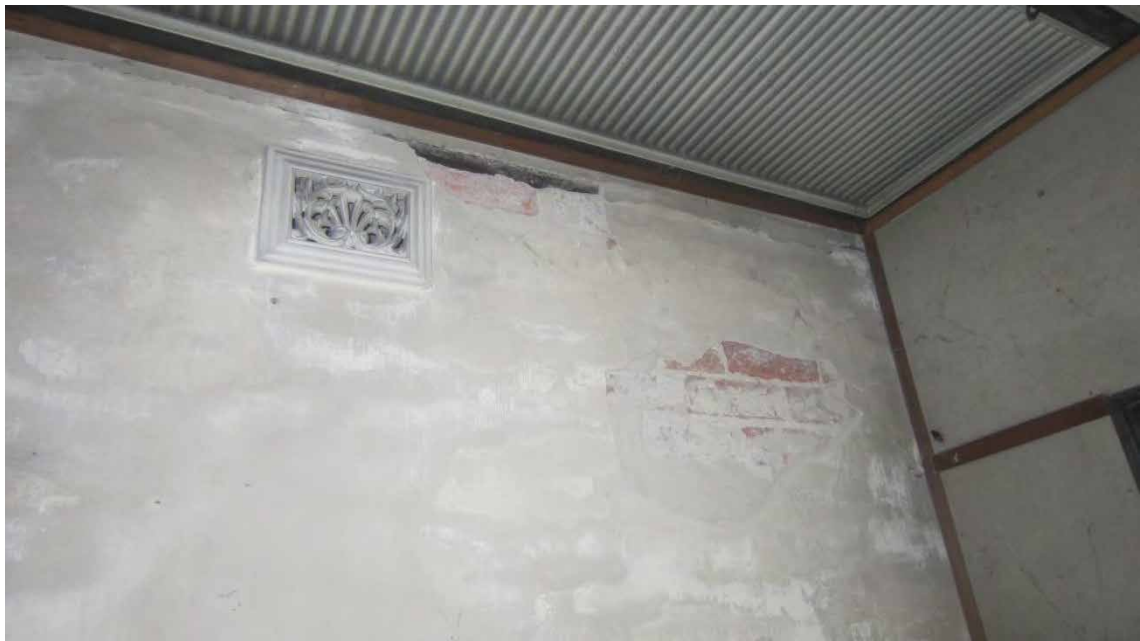
Figure 89. Southern (internal) wall of laundry, showing depleted lime plaster; note lightweight wall at right.
