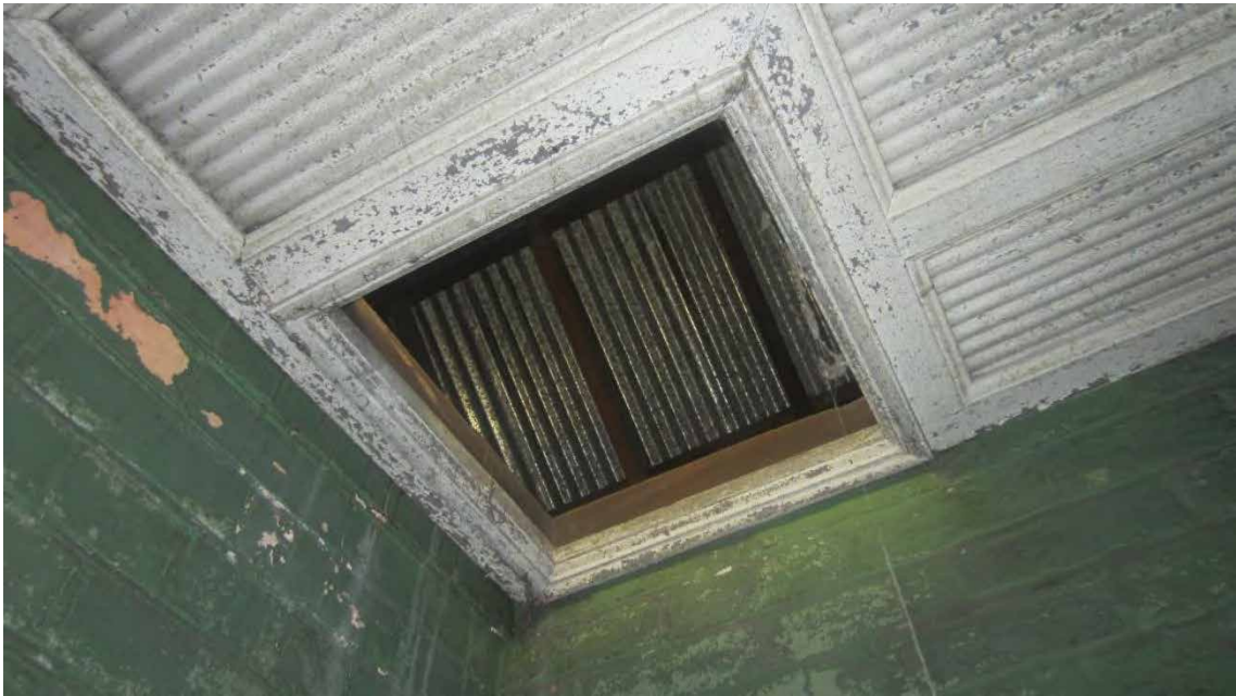
Figure 91. Roof access from hallway, showing underside of galvanised iron roof covering.
