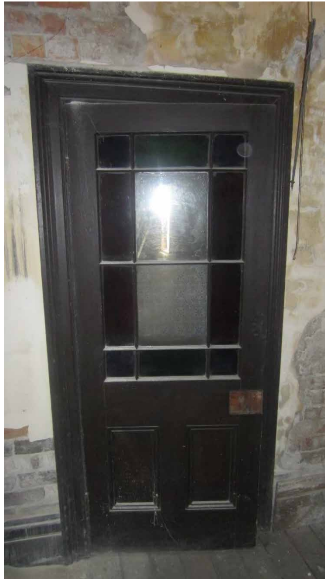
Figure 99. Door from rear hallway to dining room; note glazing colour and motifs.
