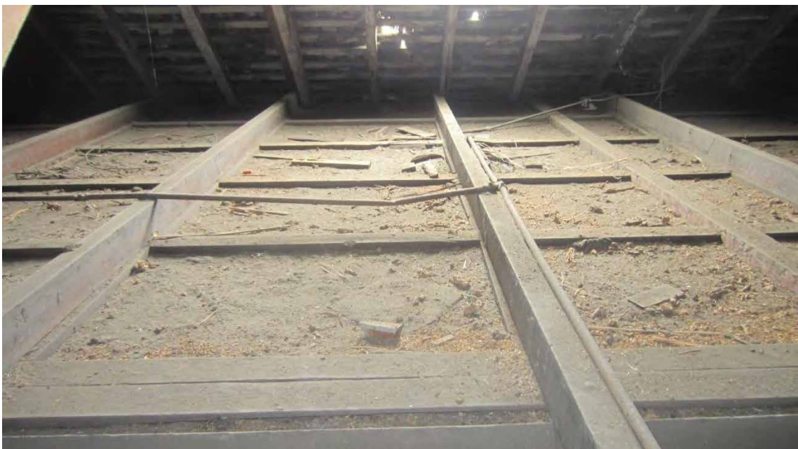
Figure 138. Roof cavity, showing top of dining room ceiling; gas light pipes still present.
