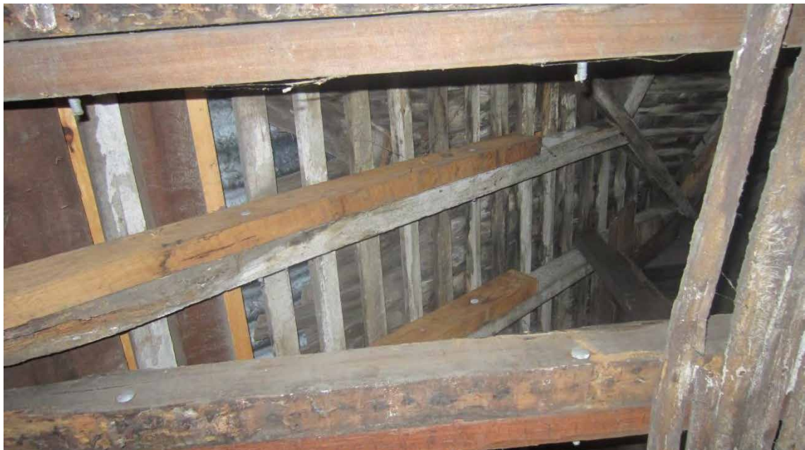
Figure 105. Depleted tongue in groove ceiling permits view of ceiling; note recent hardwood cleated to rafters and joists.
