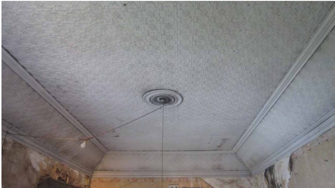
Figure 112. Pressed metal ceiling of sitting room, replacing tongue in groove ceilings and disguising amalgamation of the sitting room and north-western bedroom as originally laid out; note ceiling rose for gasolier, and later adaptation to electric light.
