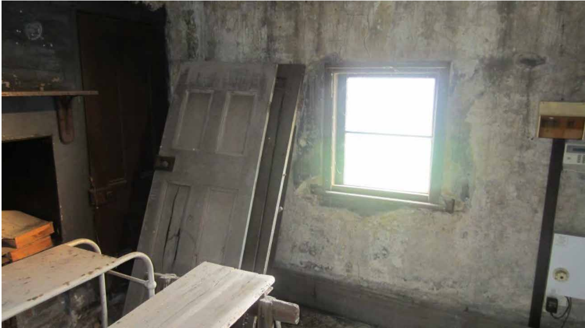
Figure 81. External door to bathroom/laundry; door leafs are from internal doorways of house.
