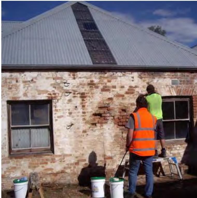
Figure 45. Repointing (with lime mortar) and desalination works in progress. Sarah Cameron via NSW Heritage Division
