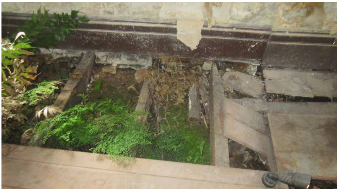
Figure 111. Plant growth in north-western corner of sitting room evinces presence of damp in sub-floor; note floor joists shaped with an adze.
