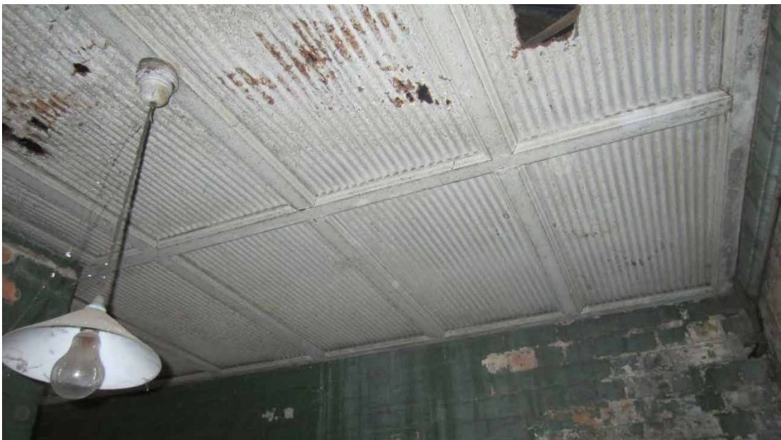
Figure 92. Hallway ceiling; note efflorescence to bricks from historic water intrusion. Light fitting is of unknown date.
