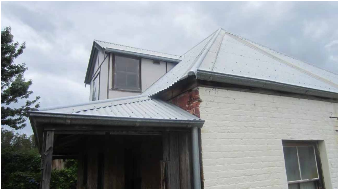
Figure 178. Missing length of gutter beneath main roof eave.
