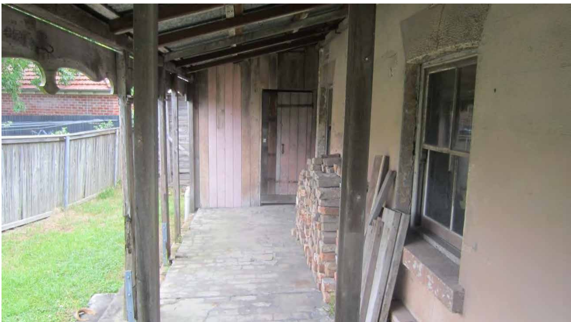
Figure 165. Southern verandah; note poor condition of verandah posts, and stockpile of bricks and timber.
