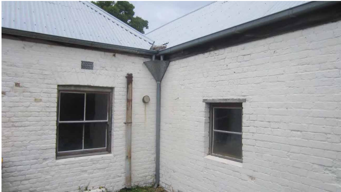
Figure 176. Limewashed walls; note redundant downpipe (left) and build-up of detritus above active downpipe (centre).
