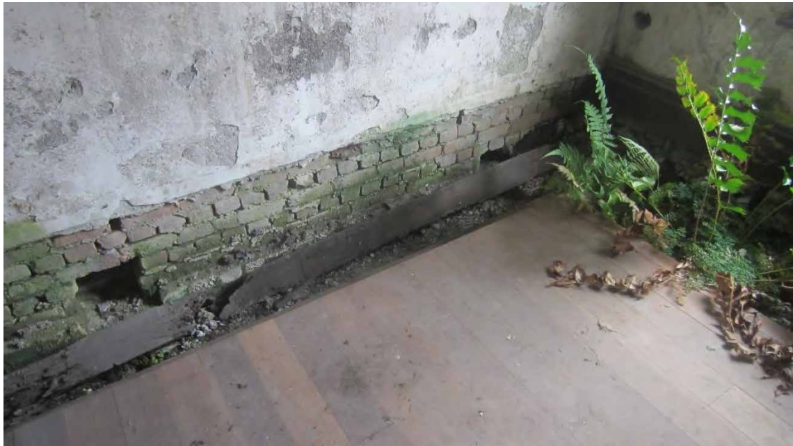
Figure 110. Western wall of sitting room; northern wall at right; note new floor, which is cannot yet be continued to wall until damp problems are addressed.
