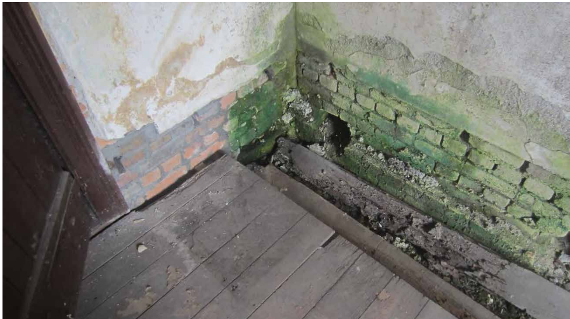
Figure 109. Sitting room, showing damp and depleted lime plaster at base of western wall (originally external); note that damage to hallway wall on left has been made good.
