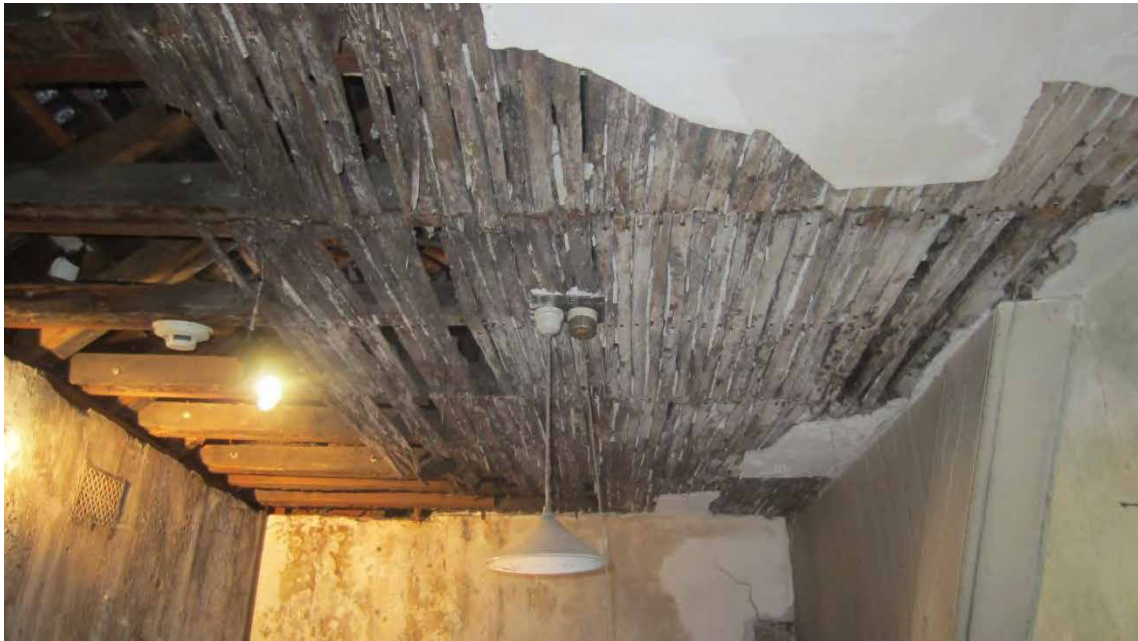
Figure 100. Ceiling of south-west bedroom, showing historic water damage.
