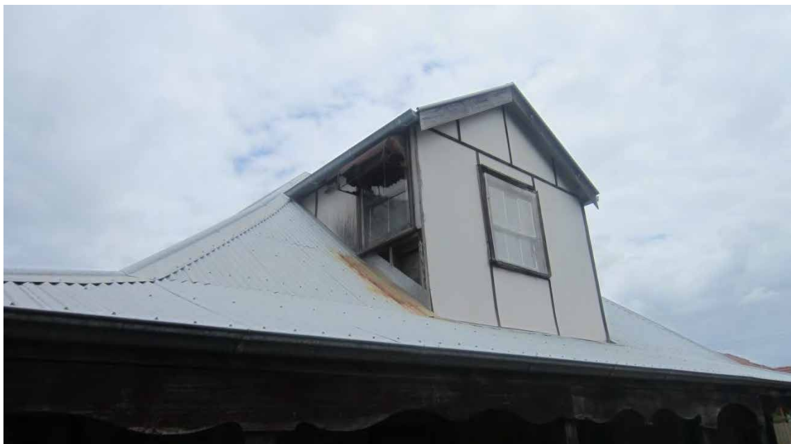
Figure 173. Corrosion marks from decaying dormer window sun canopy.
