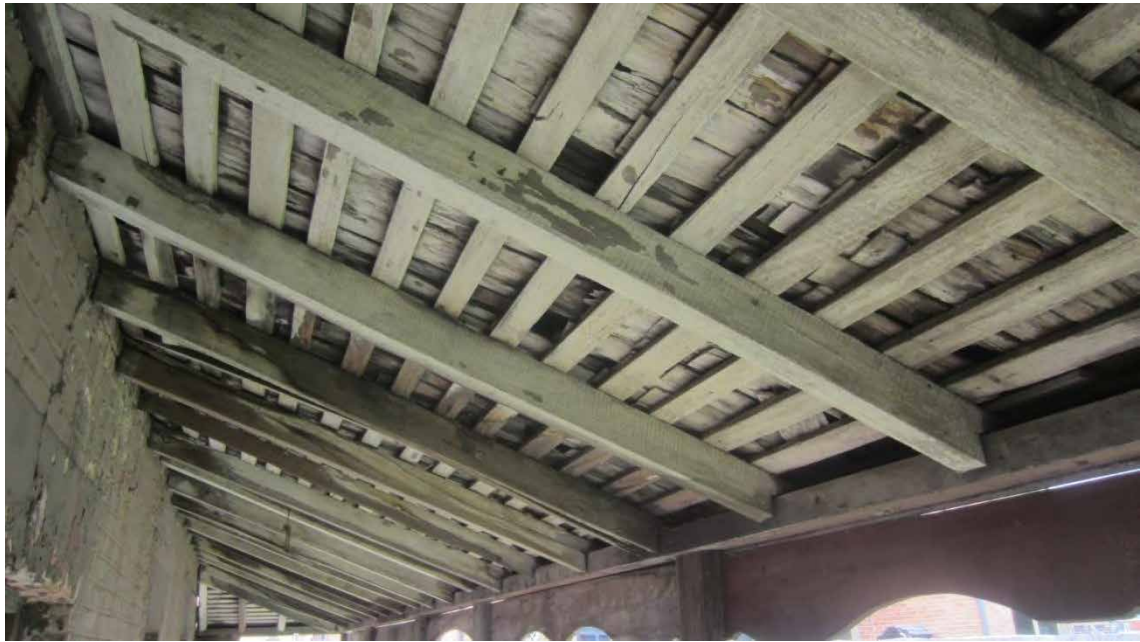
Figure 174. Timber batten and shingles of verandah roof.
