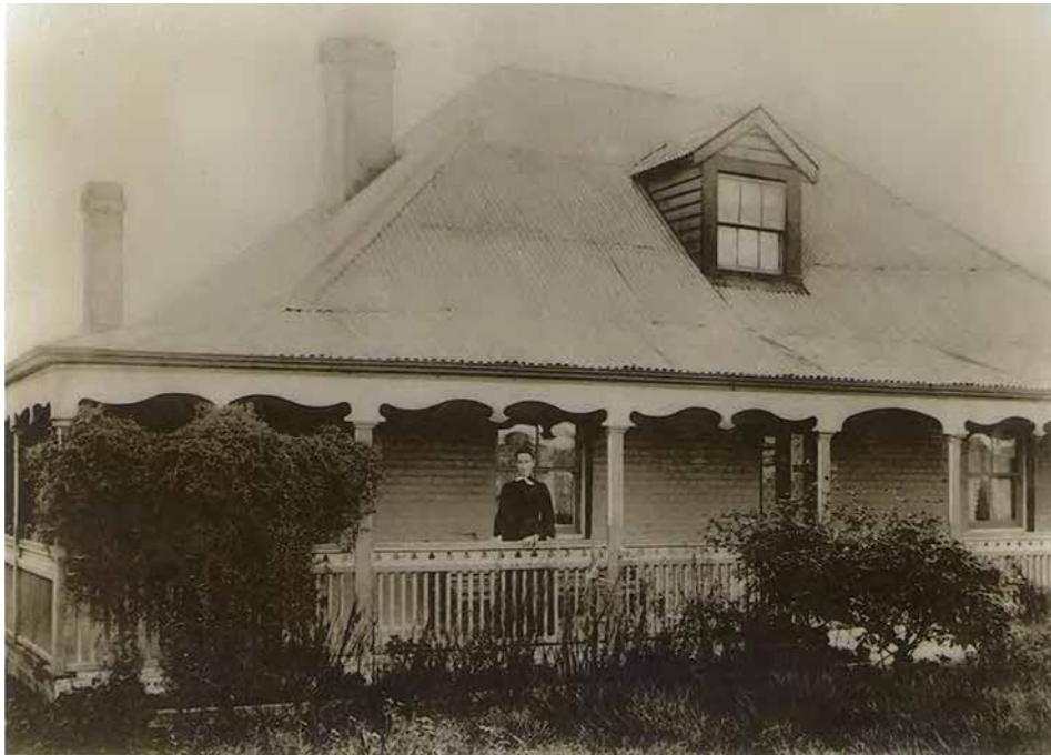
Figure 28. Photograph of the house c.1900, showing alterations and additions. The right-hand chimney has been removed, while corrugated iron has been laid over the original shingled roof. The chimney at left serves the recently-completed dining room. The verandah has been altered with the addition of a decorative balustrade and valance, replacing the originals, although the dormer window is as yet in original condition. The lady proudly standing on the verandah is Mrs Alice Little, grandmother of Naomi McCourt. Note that, due to the continued presence of roof shingles, the overlaps of the iron sheeting are unusually inconstant. The photograph was amateurishly retouched in the 1990s by a photographic laboratory to better show the profile of the chimneys. It is thought that this photograph was taken to mark the completion of the improvements undertaken by William Little. Late Mrs Naomi McCourt
