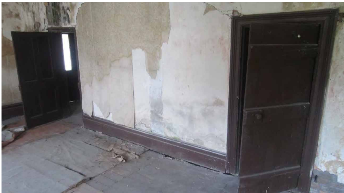
Figure 117. Contrast between door finishes; the rear of the door leaf at right, originally providing access to the former north-western bedroom later amalgamated with the sitting room to form one large room, is much more roughly finished than that of the original sitting room at left. Note short floor boards where dividing wall was formerly located.
