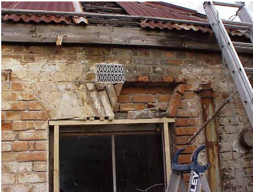
Figure 43. Conservation works to flat arch of north window. Suters Architects
