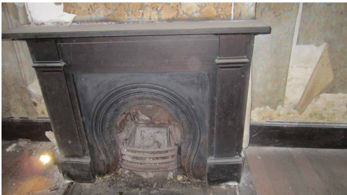
Figure 127. Fireplace; note floor repairs at right.
