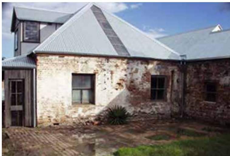
Figure 44. Looking south, showing depleted limewash and lime mortar; note brick paving.
