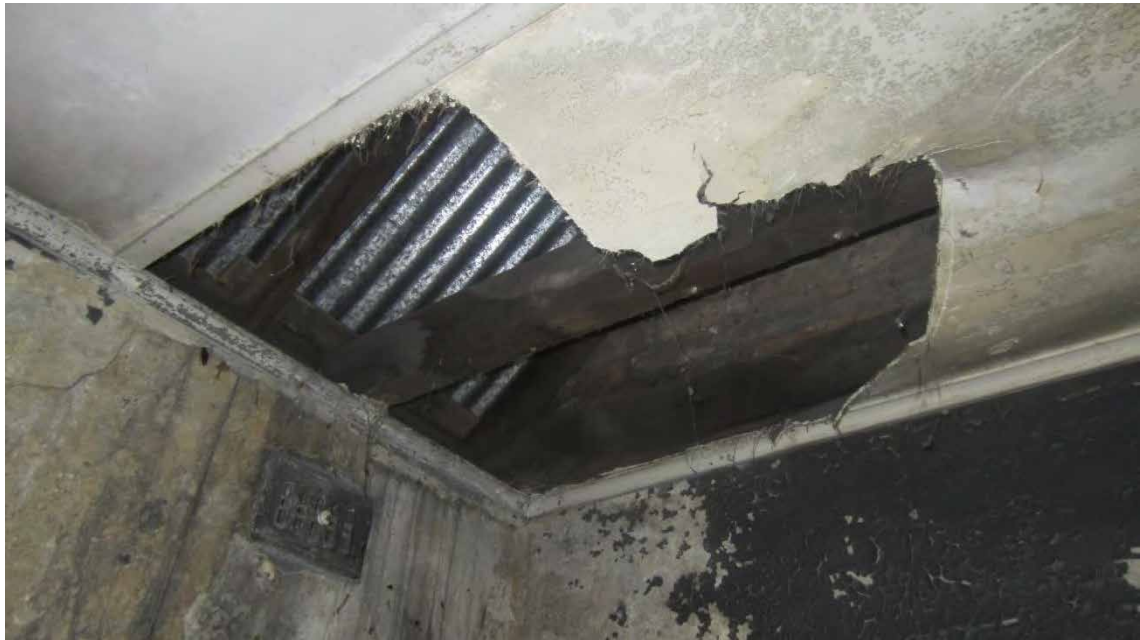
Figure 80. Water damage to kitchen ceiling.
