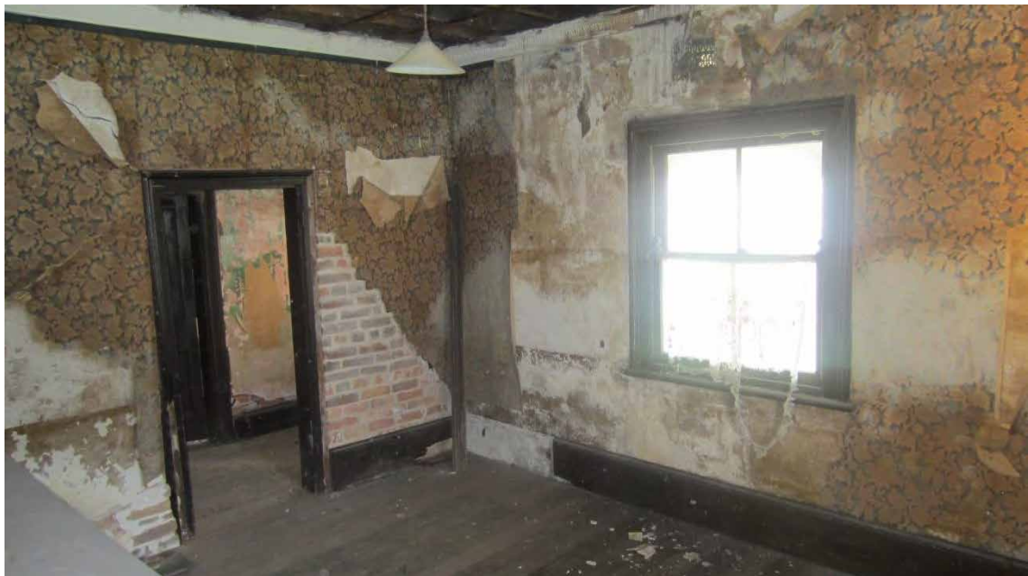
Figure 123. Looking north-east to hallway, showing partial wall reconstruction on both sides of doorway making good earthquake/ground movement damage.
