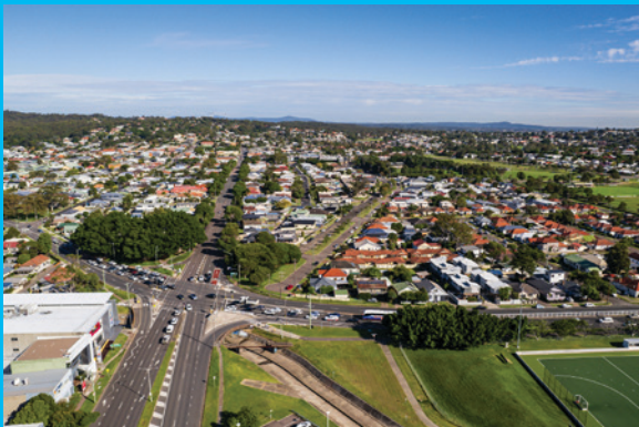
Looking east from Lambton Road and Cameron Street (Source: CN)
