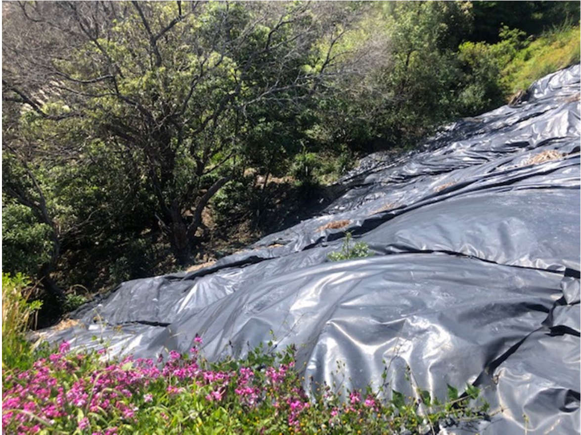
Plate 3 Area where stabilisation and remediation will occur, looking north from Memorial Drive
