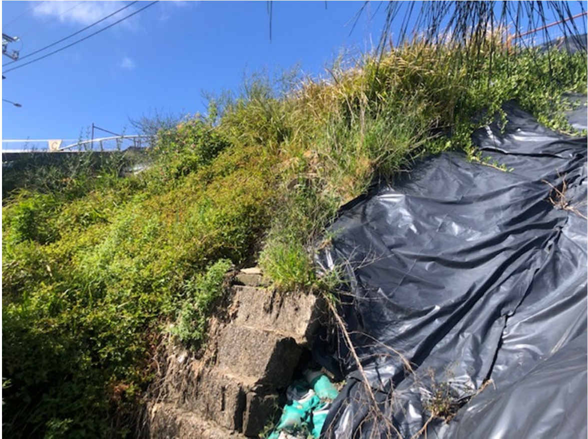
Plate 5 Location of existing stormwater pipe headwall
