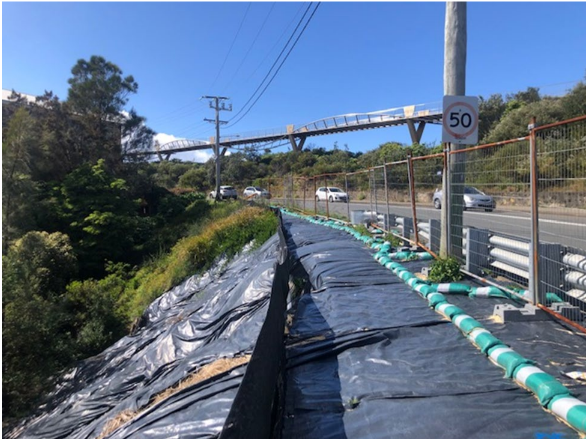
Plate 2 Top of Memorial Drive looking east with temporary slope stabilisation measures
