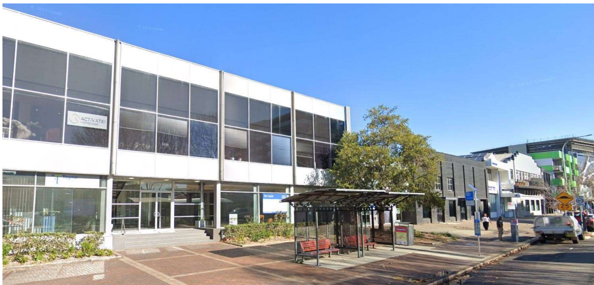
Figure 91: 239 King Street, Newcastle facing west (Source: Google Streetview)
