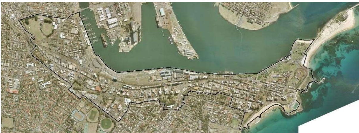
Figure 25: Aerial photograph of land in Newcastle City Centre boundary, August 2004 (Source: CN GIS)
