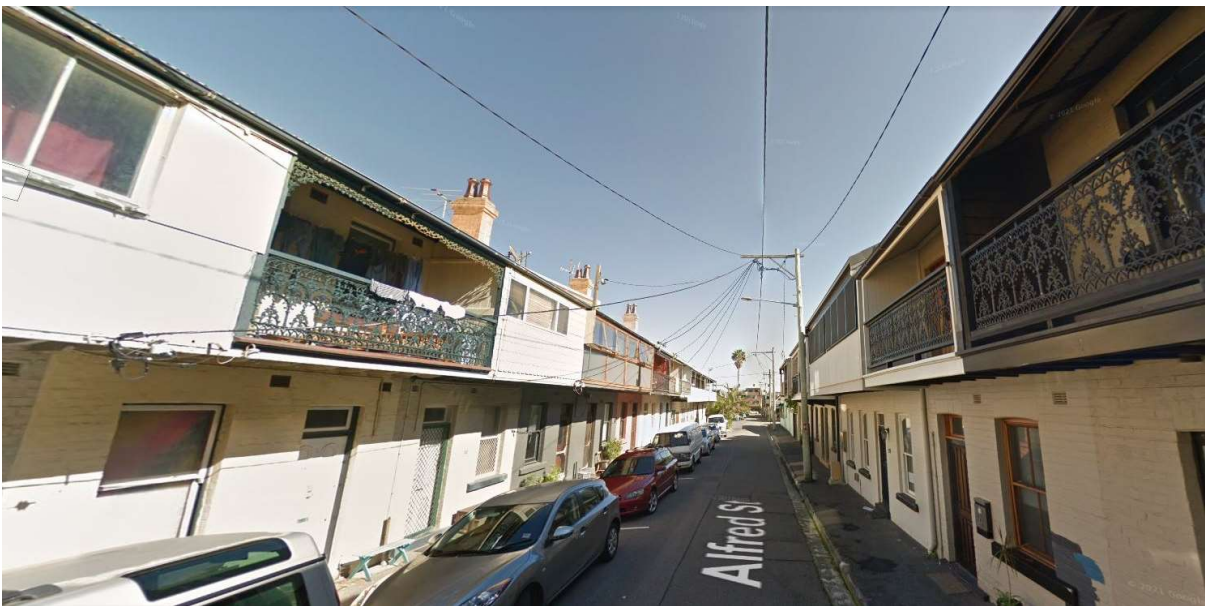
Figure 32: 8 and 11 Alfred Steet, Newcastle East facing west (Source: Google Streetview)
