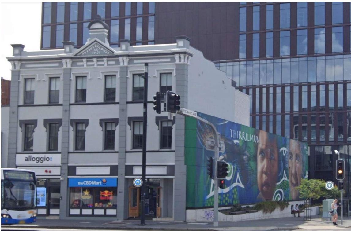
Figure 136: 840 Hunter Street, Newcastle West (Source: Google Streetview)
