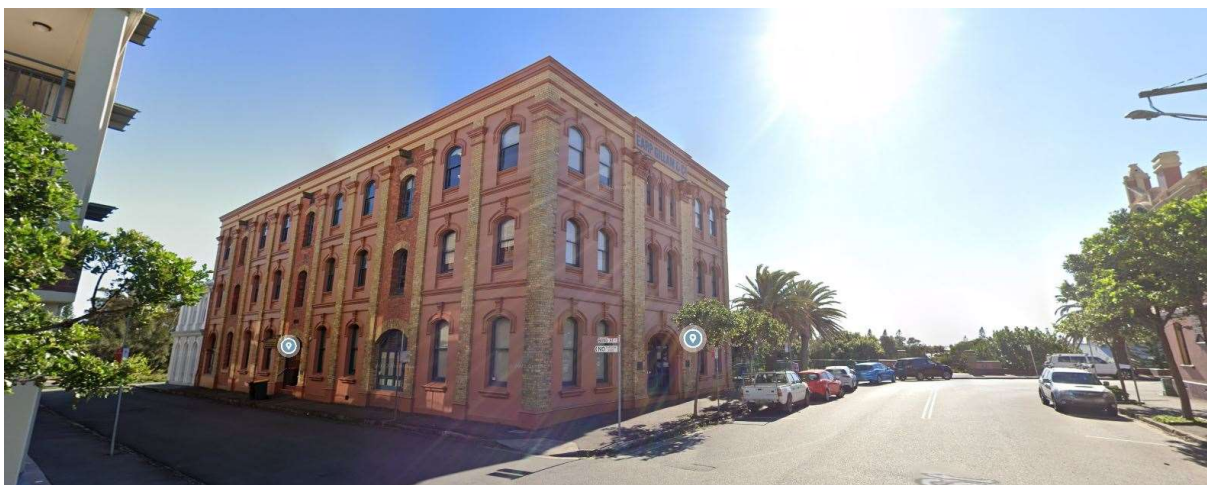
Figure 30: Earp Gillam Bond Store at 16 Telford Street, Newcastle East (Source: Google Streetview)
