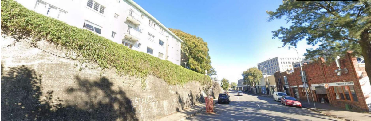
Figure 86: 199 and 218 King Street, Newcastle facing west (Source: Google Streetview)
