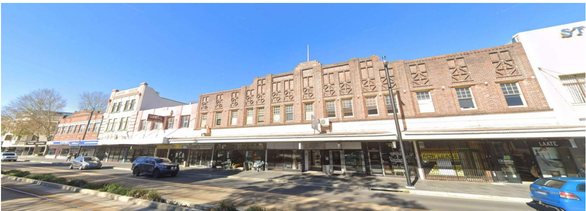
Figure 87: 269 to 283 Hunter Street, Newcastle facing east (Source: Google Streetview)
