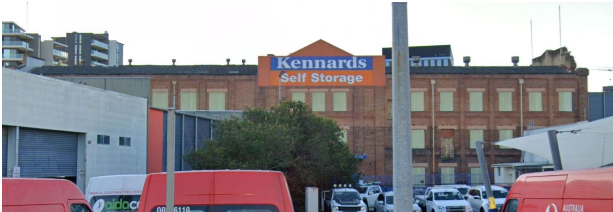
Figure 137: 904-908 Hunter Street, Newcastle West (Source: Google Streetview)
