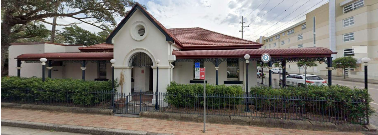
Figure 85: Fanny's Tavern at 311 Wharf Road, Newcastle (Source: Google Streetview)
