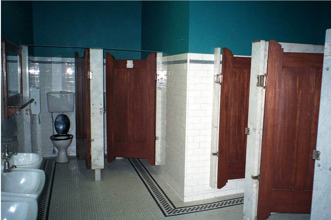
Figure 25: Ground Floor Ladies Toilets in 2001. If the use of the space needs to change to make loading and kitchen areas more viable, then consider re-using some of the original fittings in the new WC facility. An archival record should also be made of the space prior to change.
