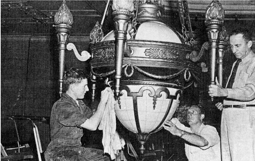
Figure 21: Chandelier Cleaning (NCC Photo)
