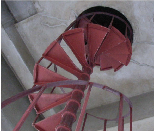
Figure 23: Steel Spiral stair in NCH Clock Tower 2008
