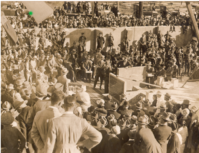
Figure 1. Laying of Foundation Stone by Sir Dudley de Chair 20 April 1928 NC/A
